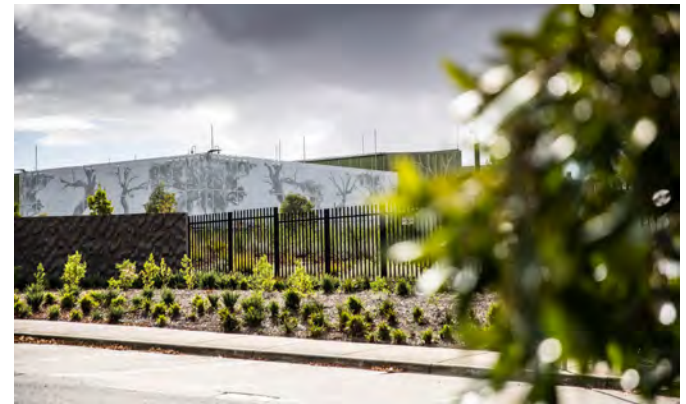
Precedent image from DS-09 showing a TPSS. Brunswick East, Australia. Image Credit: Beca .
