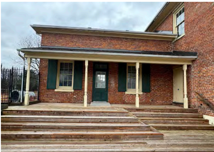
North elevation illustrating the porch, the wood deck, entrance and two flanking windows. The filled-in right apron wall suggests that a door may have previously existed at this location.
