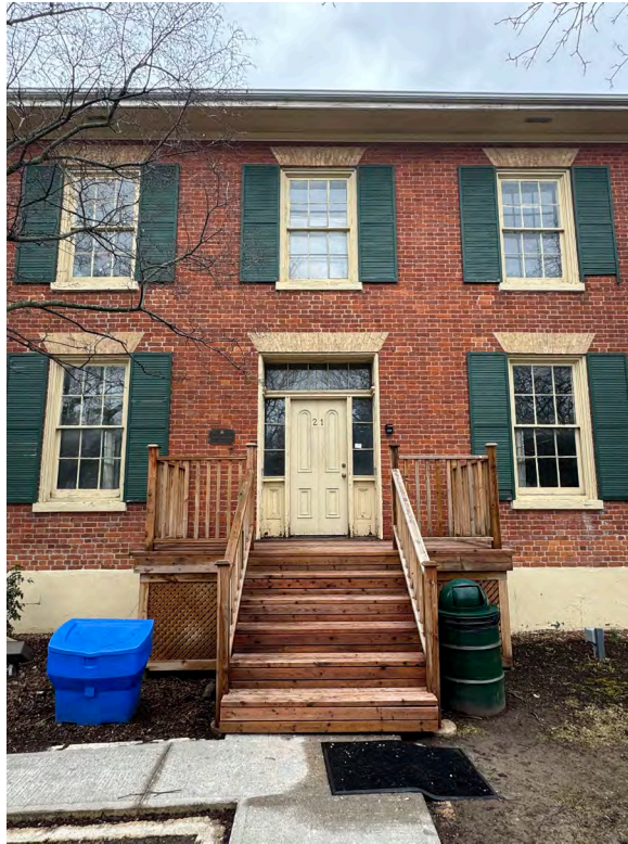
View of the main facade (west) illustrating its composition of 3 bays and its central door, and the platform named “verandah”.
