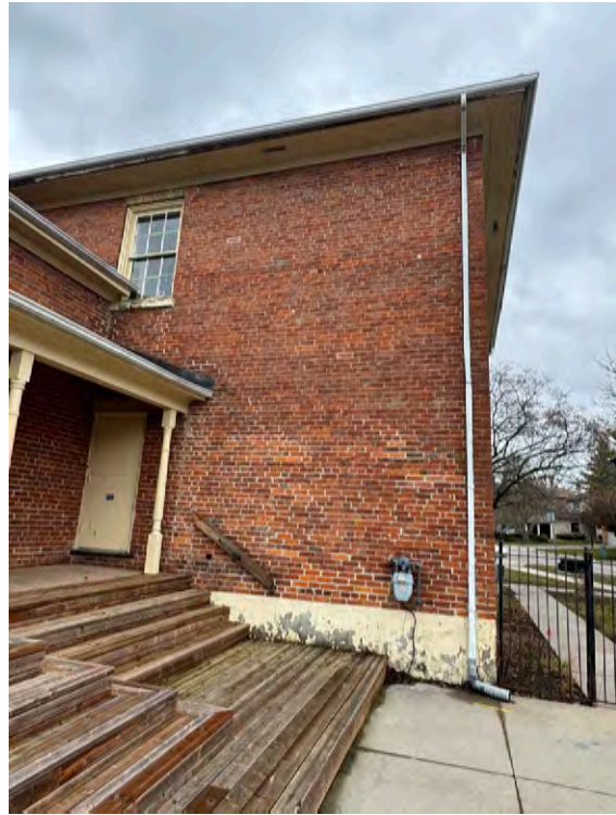
Detail of the recent wood deck leading to the porch.
