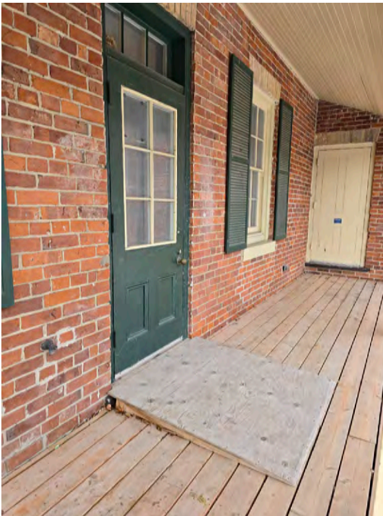
Detail of the wood door that has been replaced in the 1980's under the porch. The wood door on the background is original.
