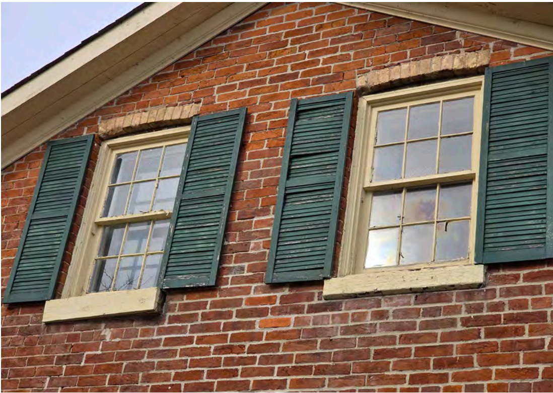
Detail of the top windows located on the east elevation. Wood window sills were replaced and shutters were added in the 1980's.
