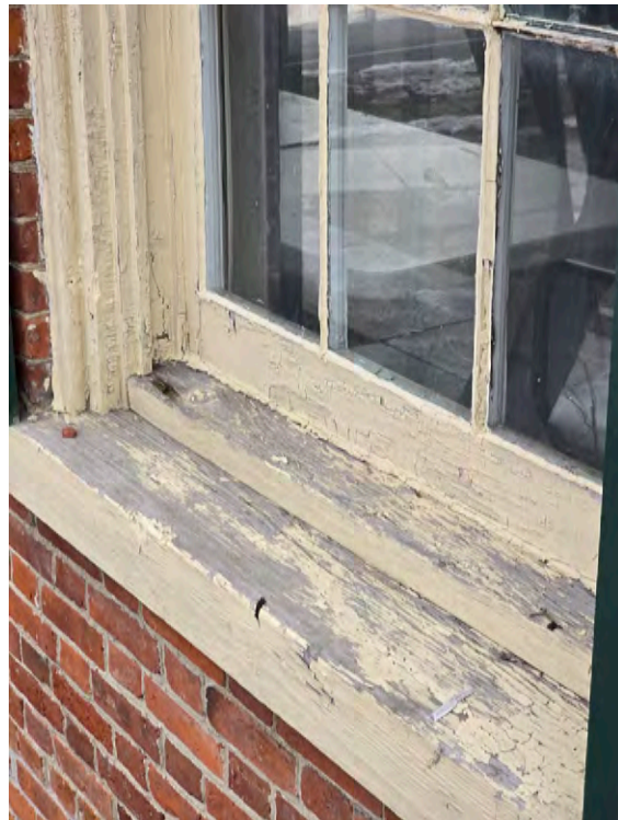
Detail of the wood window sill located under the porch.
