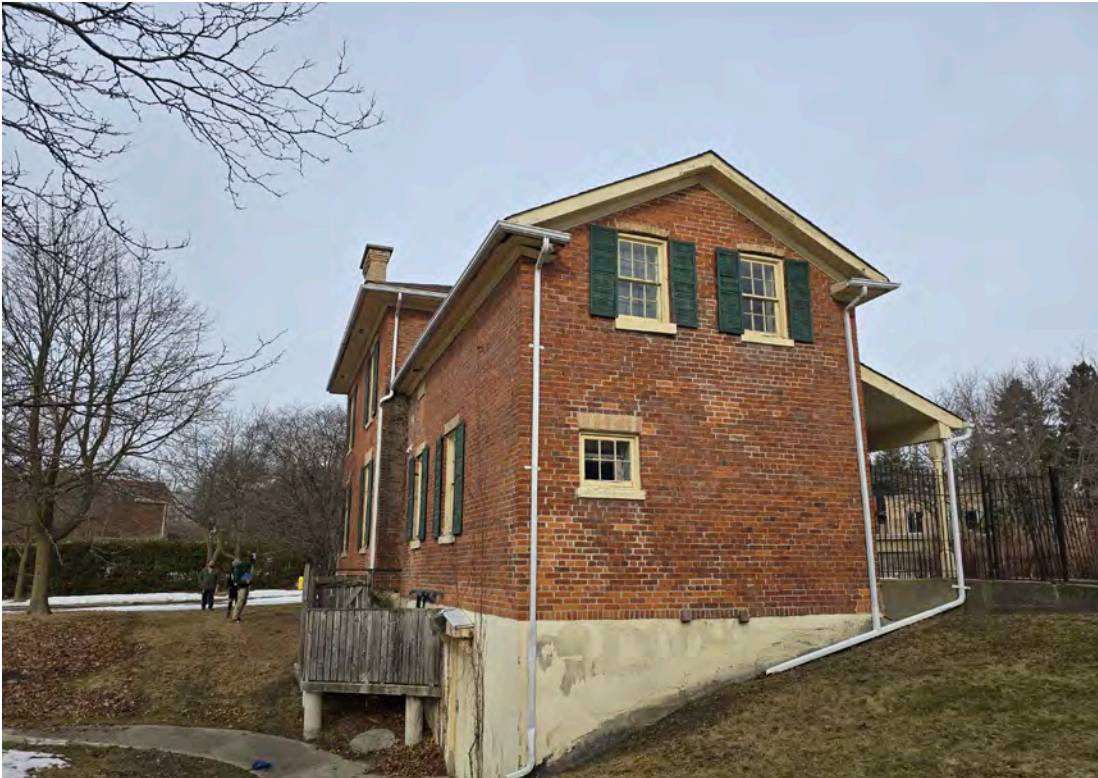
View of the east elevation.
