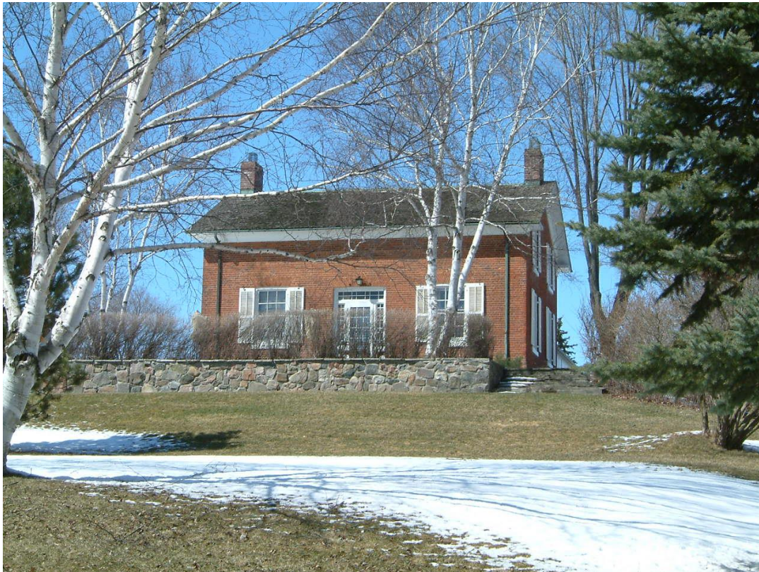
Figure 2. 5800 King Vaughan Road South Elevation (City of Vaughan, 2005).
