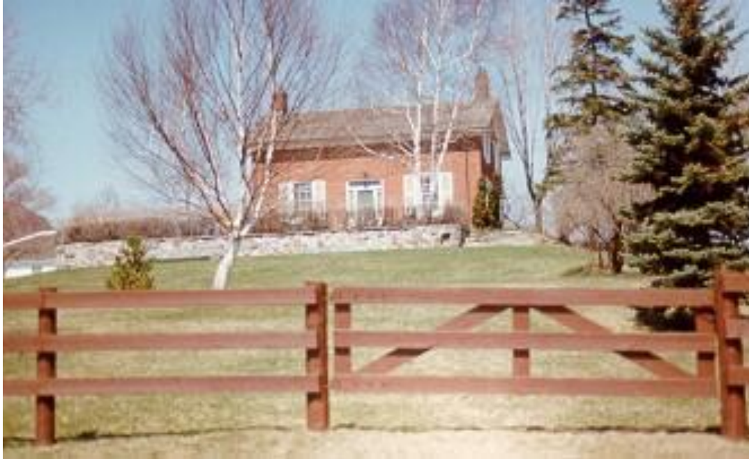
Figure 1. 5800 King Vaughan Road South Elevation (City of Vaughan, 2001).
