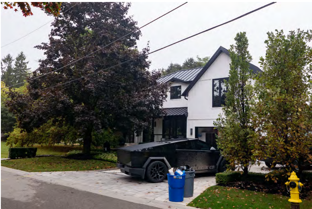
Figure 14: Southeast view of the east elevation showing the hipped roof section left of the gable (CBCollective 2025).
