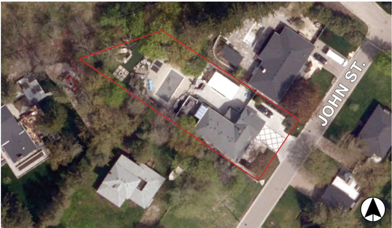
Figure 2: Aerial photograph from 2024 showing the subject property (red outline) at 22 John Street (York Region, CBCollective 2025).
