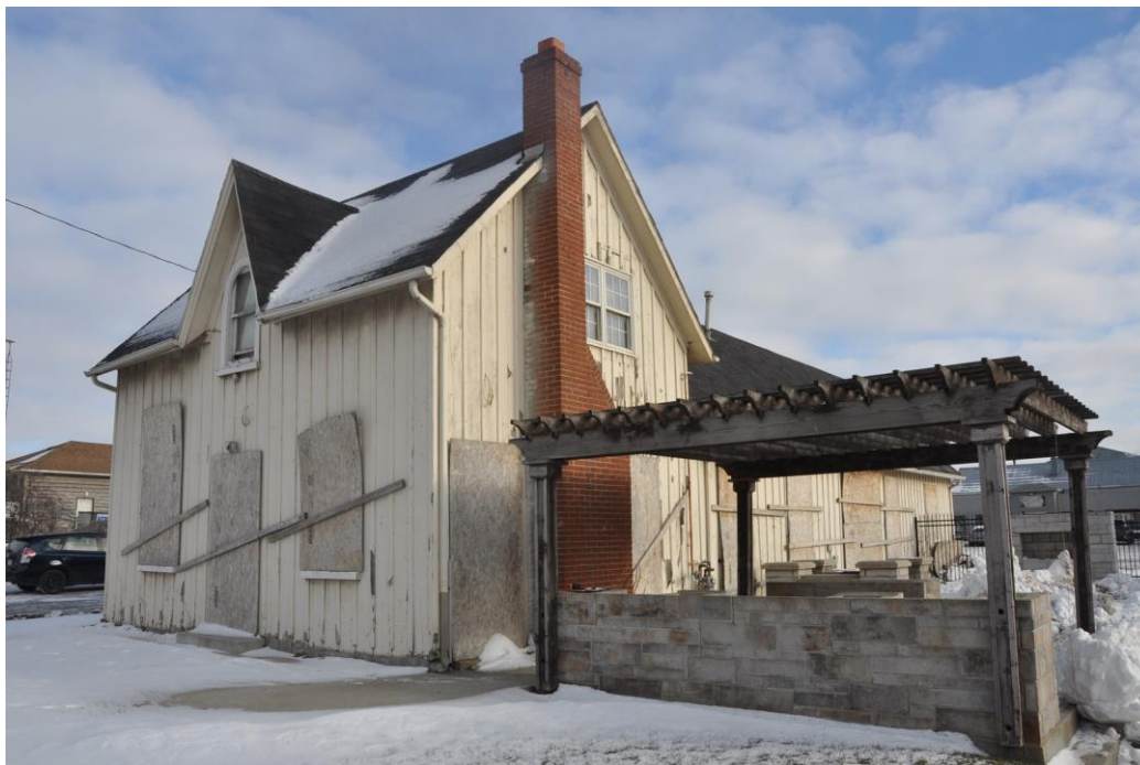
4.1.5.1.B - Existing view from southwest
