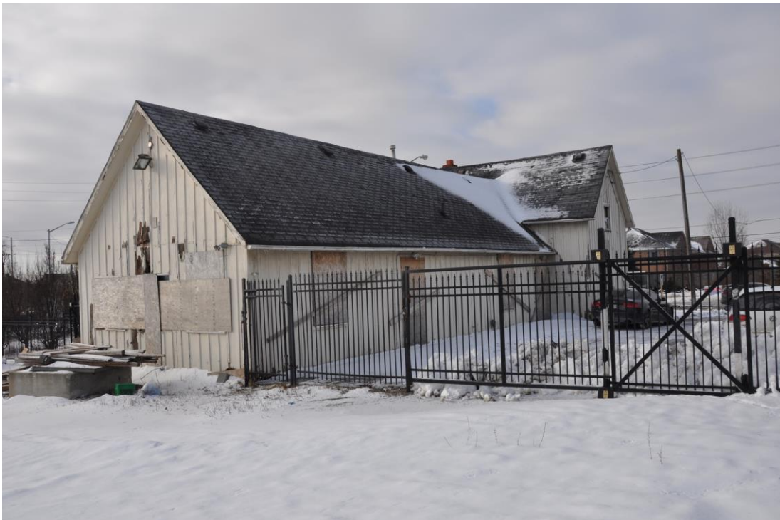
4.1.5.1.F - Existing View from Northeast
