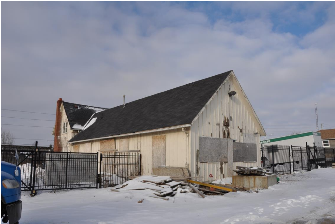
4.1.5.1.D – Existing View from Southeast
