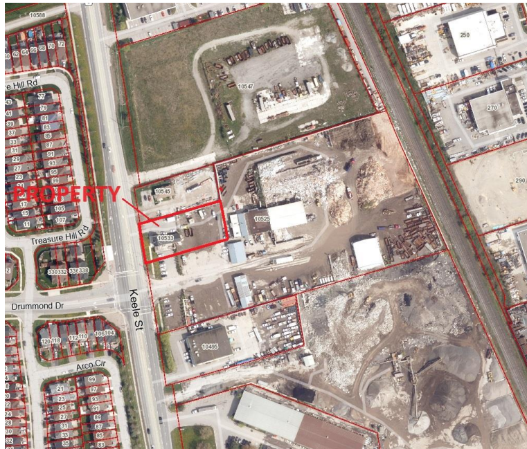
4.1.1.A - Aerial Photograph – Property Context
