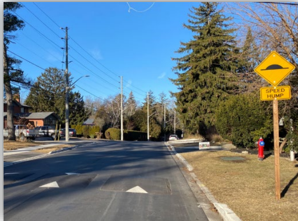
Asphalt Speed Cushions
