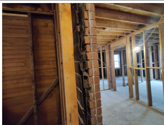
Figure 23. Surprise! Underneath the brick veneer is the previous cladding of untapered clapboard—very much old style.
