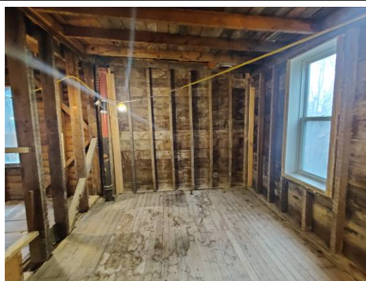
Figure 26. Kitchen tail, looking north. Note that walls are of sheathing, not clapboard. There may have been a different exterior finish. Board and batten was a common siding on kitchen tails.
