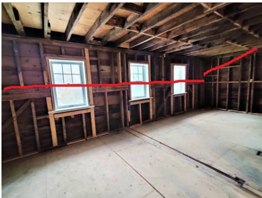
Figure 30. The red line on the left follows the top of the original header beam. It has been cut to fit the windows. The red line to the right follows the line of the original gable header. Everything above these lines was added—most likely at the time of the brick veneer installation.
