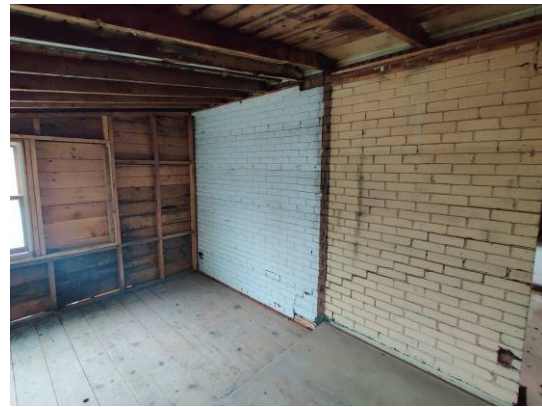
Figure 40. Settlement cracking, second floor rear wall.
