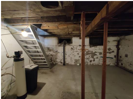
Figure 11. The basement extends under the original house, and additions are unexcavated. This view is from the middle of the main body of the house to the northeast corner. A steel post and timber beam have been installed to support the original heavy timber summer beam, which is also supported by a second steel post.
