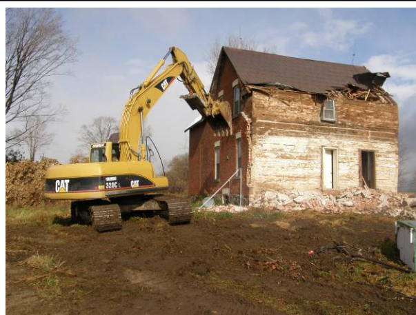
Figure 45. Stripping brick veneer from another log house, this one in Stroud. It's fast work for a skilled operator. Photo by Vic Snow.
