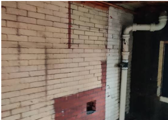
Figure 41. Settlement cracking second floor rear wall.
