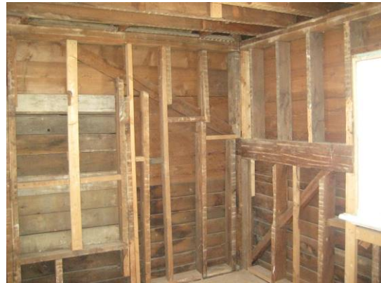
Figure 32. On the left, you can see filled-in original window in the south gable end. Note that its head is higher than the header beam to the right.
