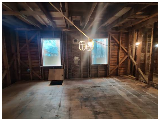
Figure 25. Northeast corner, with kitchen tail to the right. The mortised bracing of the corner post is very evident here.
