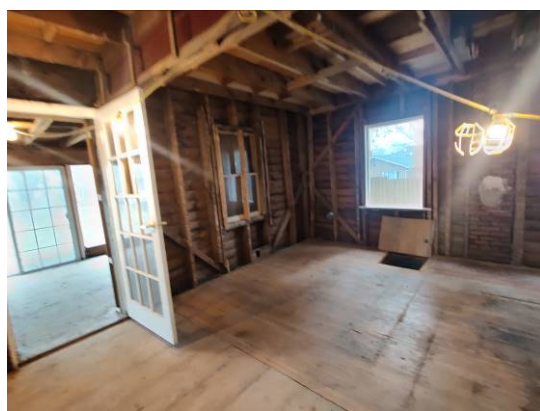
Figure 24. Northwest corner of the ground floor. The diagonally-braced corner post and door post are evident, as is the clapboard siding on both exterior walls.
