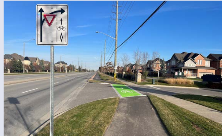
Weston Road sidewalk and cycle tracks
