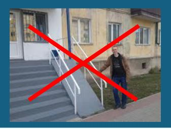
Maximum Slope of Ramp Under the Current IDS (1:15)
