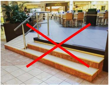
Recommendation 8: The Maximum Slope of Ramps should be 1:20
