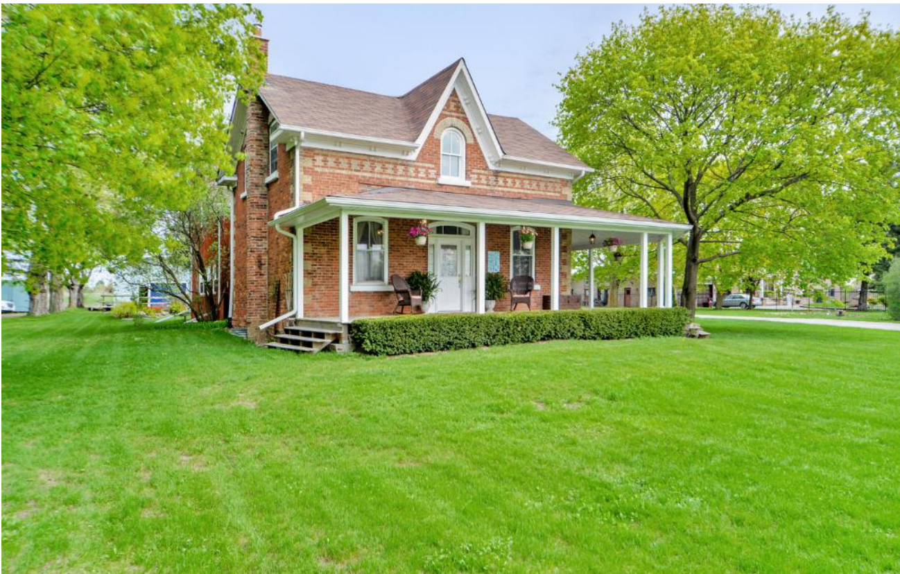
Figure 6. 6120 King Vaughan, South and West Elevation (2013 Listing. https://tours.virtualgta.com/public/vtour/display/109751?a=1#!/ )
