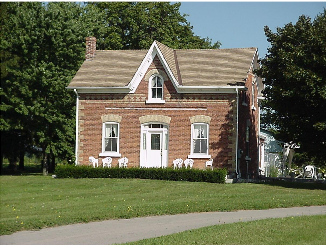
Figure 2. 6120 King Vaughan Road, South Elevation (City of Vaughan, 2005).
