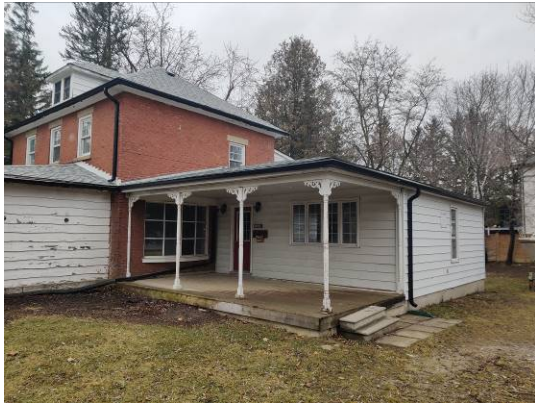
Figure 17. The south addition is relatively recent and the porch is constructed with dollar store posts and gingerbread. This has no heritage interest.
