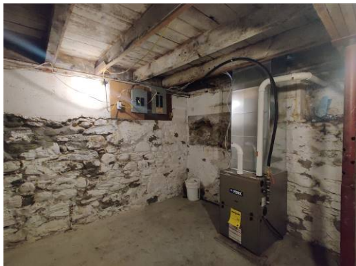
Figure 12 looking to the southeast corner. Note lower foundation of fieldstone & concrete above.
