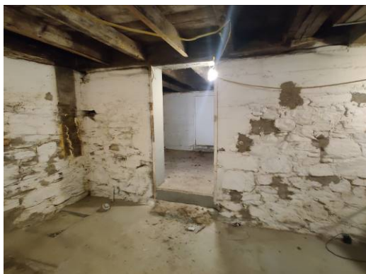
Figure 13. Looking into foundation of the tail, with the exterior door beyond.
