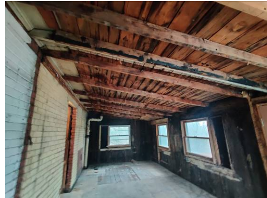
Figure 20. Standing in the east room on the second floor, looking north. Because the brick has already been installed on the main house, we know that this room is a later addition.
