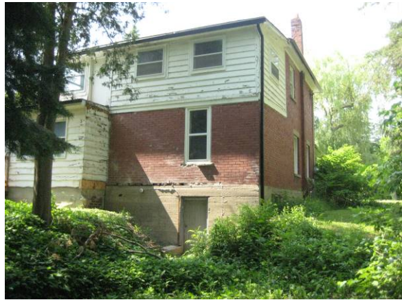
Figure 2. North east view.
