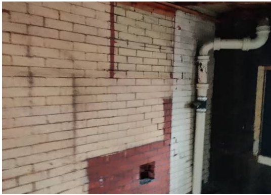
Figure 41. Settlement cracking second floor rear wall.
