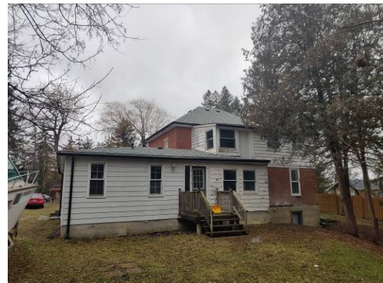
Figure 22. Rear (east) side of the house. We know from the foregoing that all of the “clapboard” bits—wood or aluminum—were constructed after the main body of the house.
