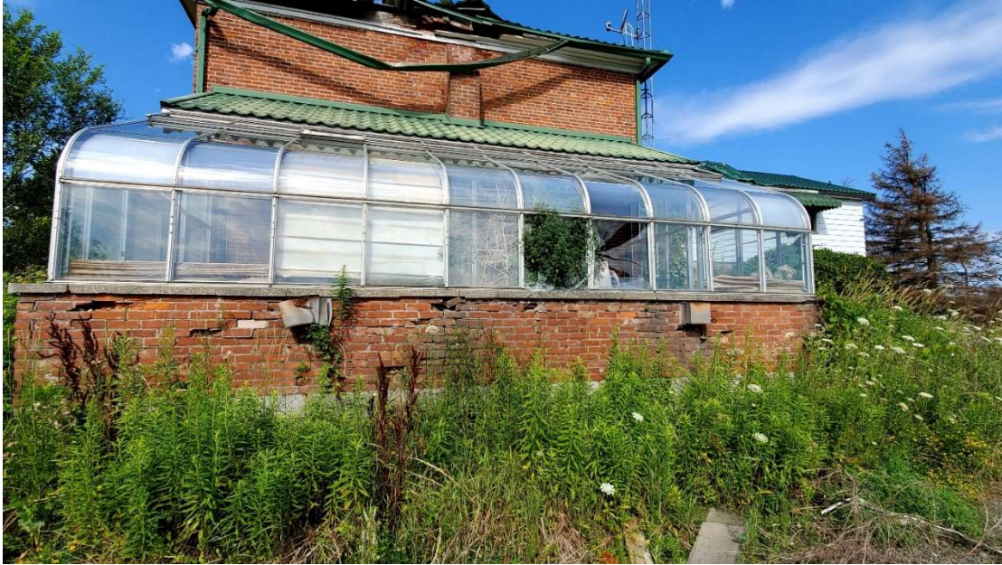
Pic. 8: Eastview showing disintegrated Masonry Wall, Vegetation growth in the Greenhouse with Broken Panes
