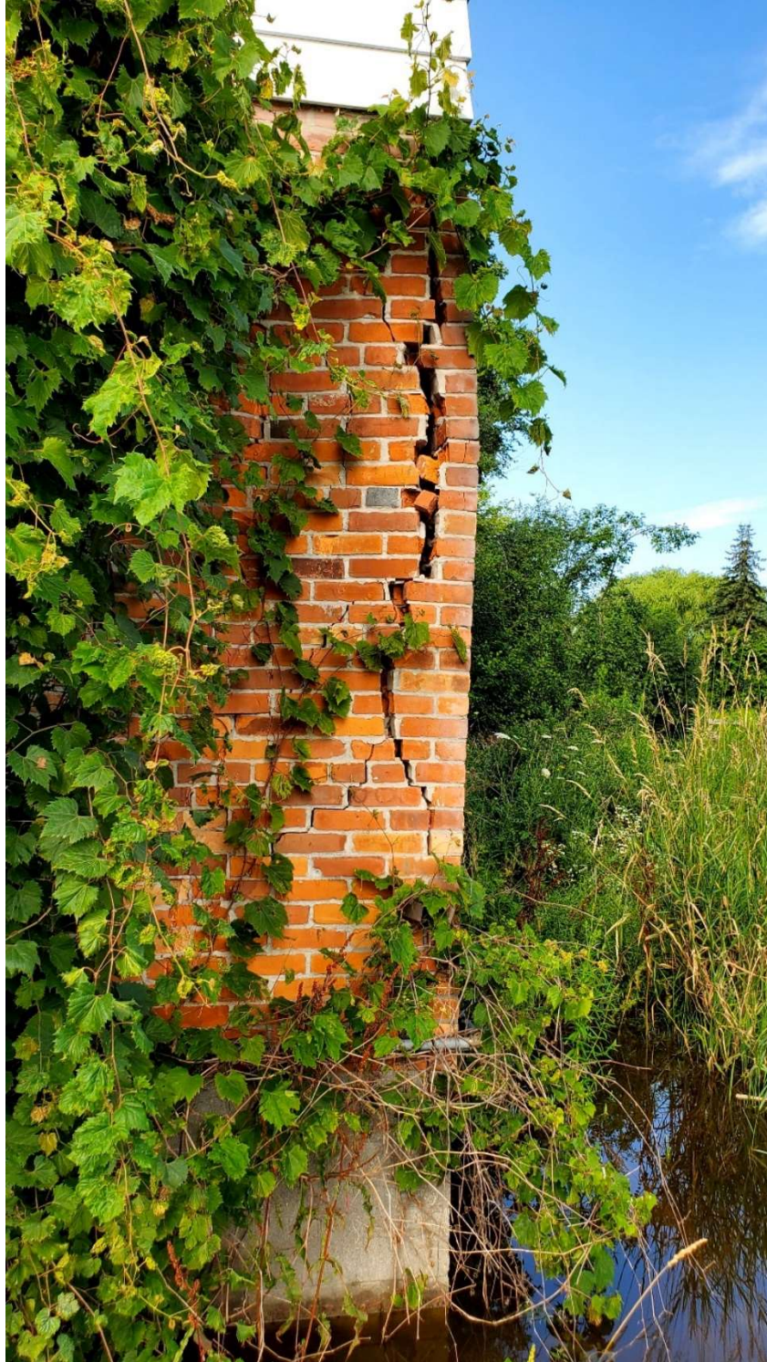
Pic. 10: Wide and Long Vertical Crack on the Northside House Addition and Water Pool Outside
