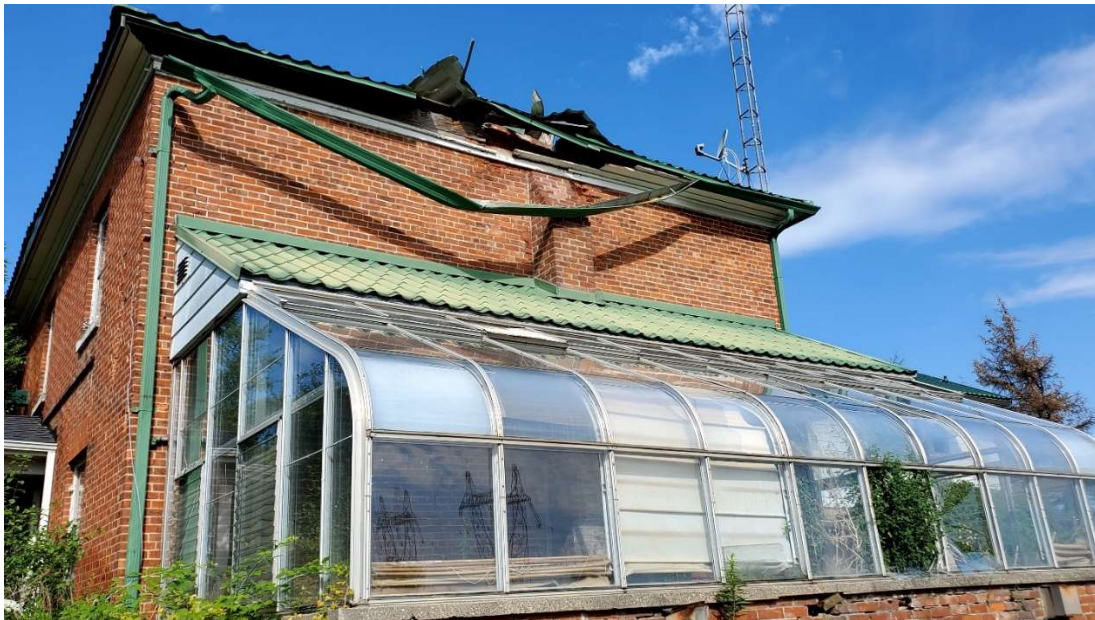
Pic. 7: Eastside View of the House showing Damaged Roof at Broken Chimney and Greenhouse Addition
