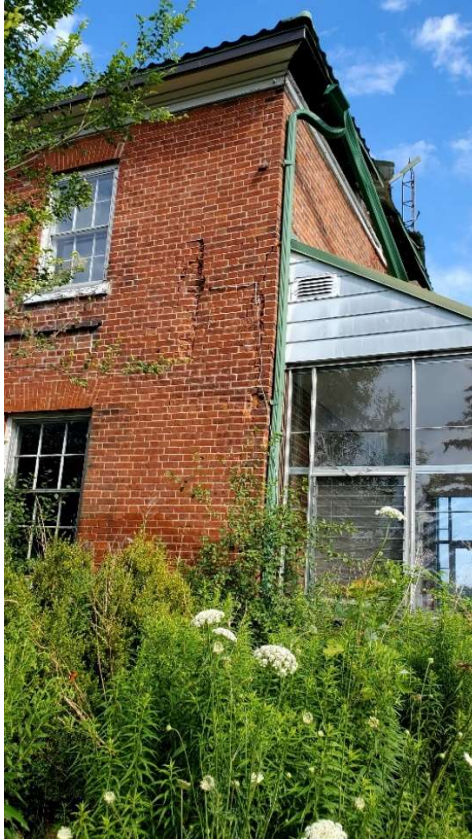
Pic. 6: Cracks and Damage on the Southside Masonry Wall of the House
