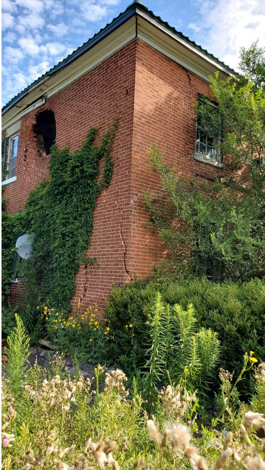
Pic. 5: Southwest view of the House-Cracks and Damage in the Load-bearing Masonry Wall
