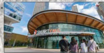
SmartVMC Bus Terminal
