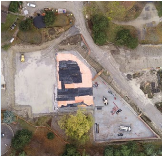
Gallanough Park Stormwater Management Facility
