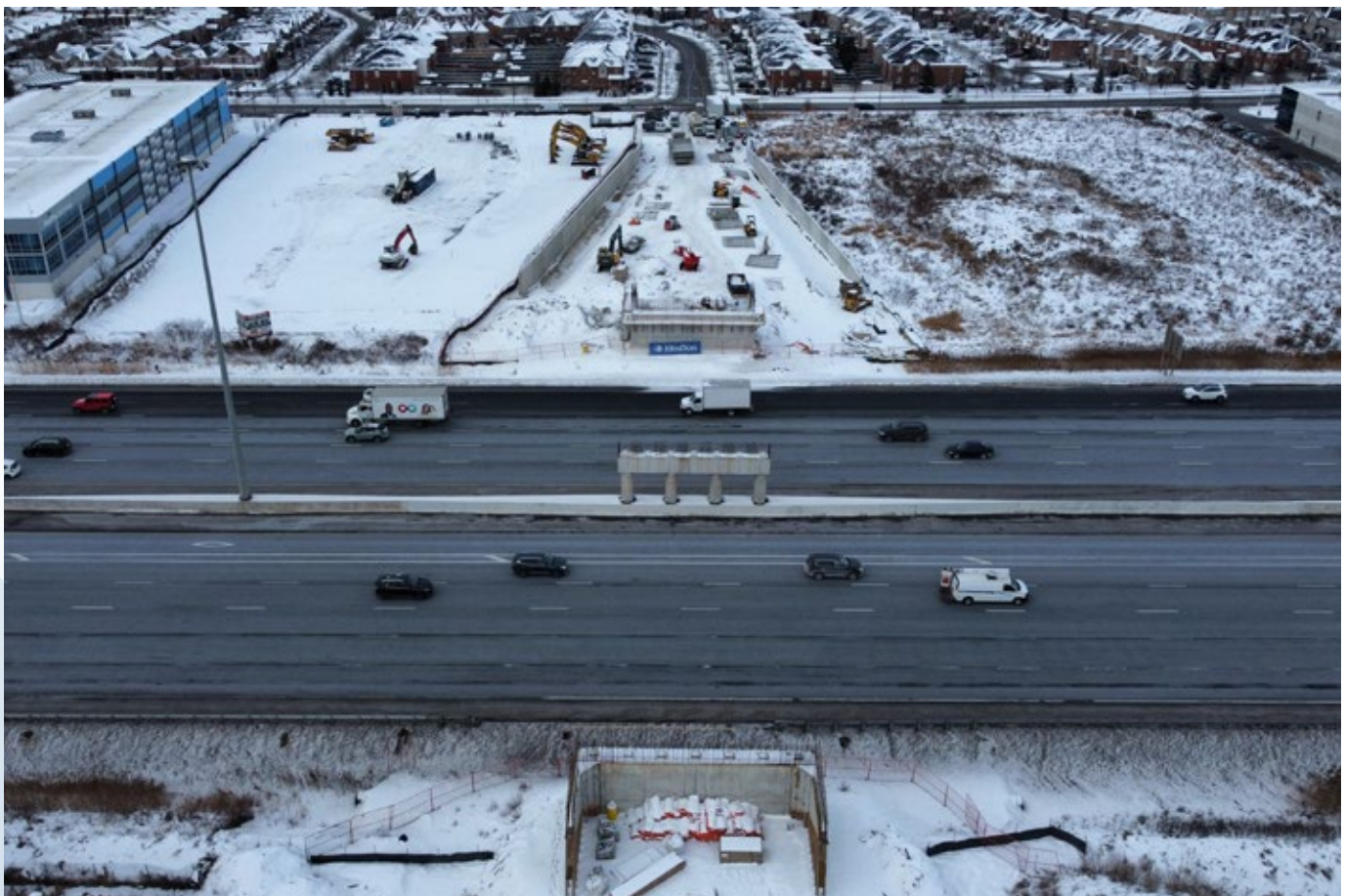
Canada Drive - America Avenue bridge construction
