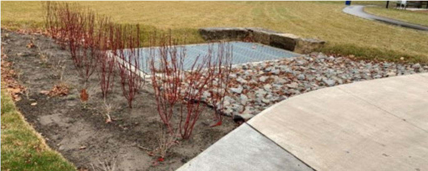
Gallanough Park stormwater management facility
