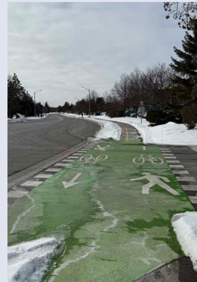
Courtland Avenue multi-use path
