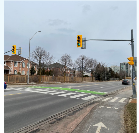
A new pedestrian crossing was built at St. Elizabeth Catholic High School
