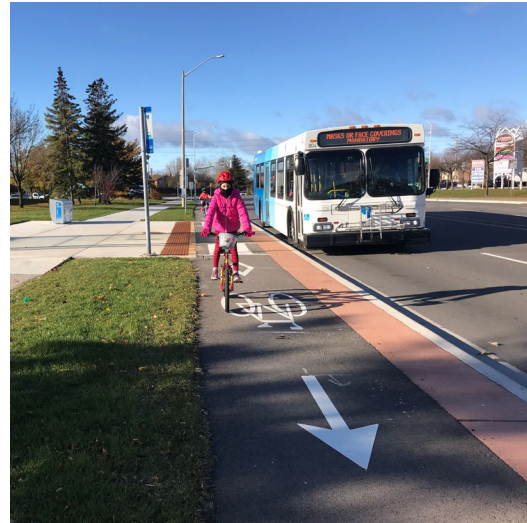
City's first retrofit cycle tracks on Clark Avenue
