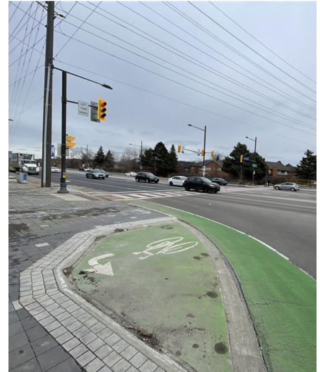
Bathurst and Centre Rapidway Project (cycle tracks and pedestrian clearways)
