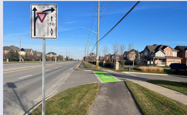
Weston Road sidewalk and cycle tracks
