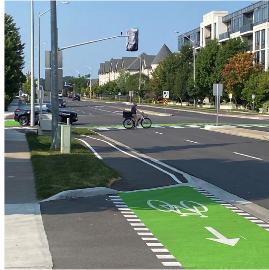
New cycle tracks on New Westminster Drive from Clark Avenue to Bathurst Street were completed
