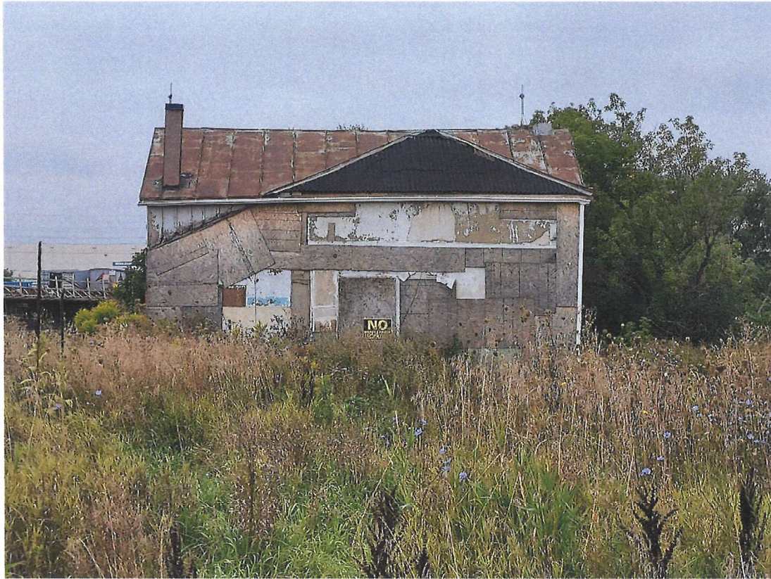
Photo 1 - View of building from the East
