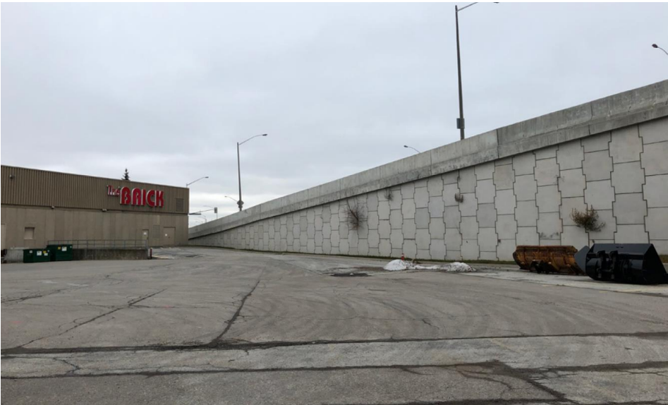
Figure 3 – Looking East Toward Highway 400 from the Site
