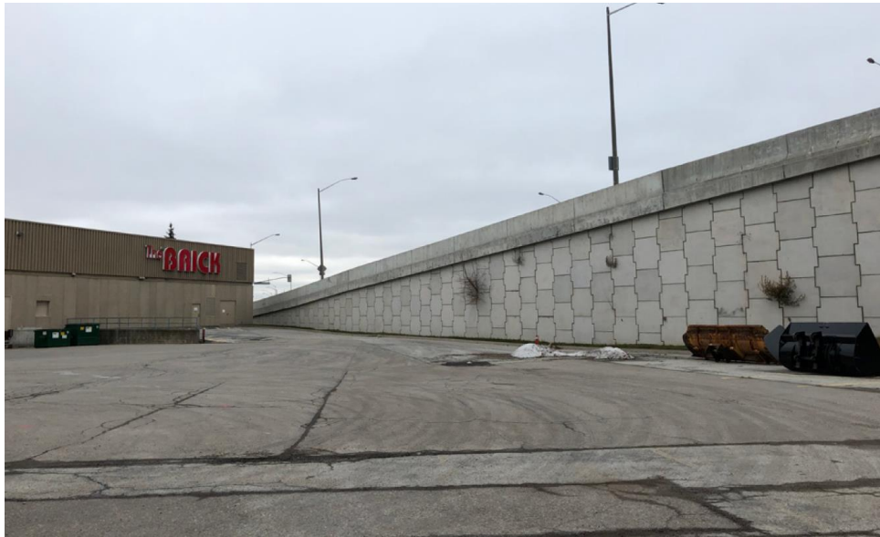
FIGURE 4 – Looking East Toward Highway 400 from the Site
