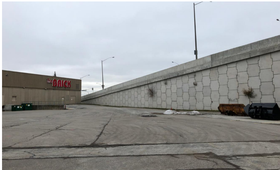
FIGURE 4 – Looking East Toward Highway 400 from the Site
