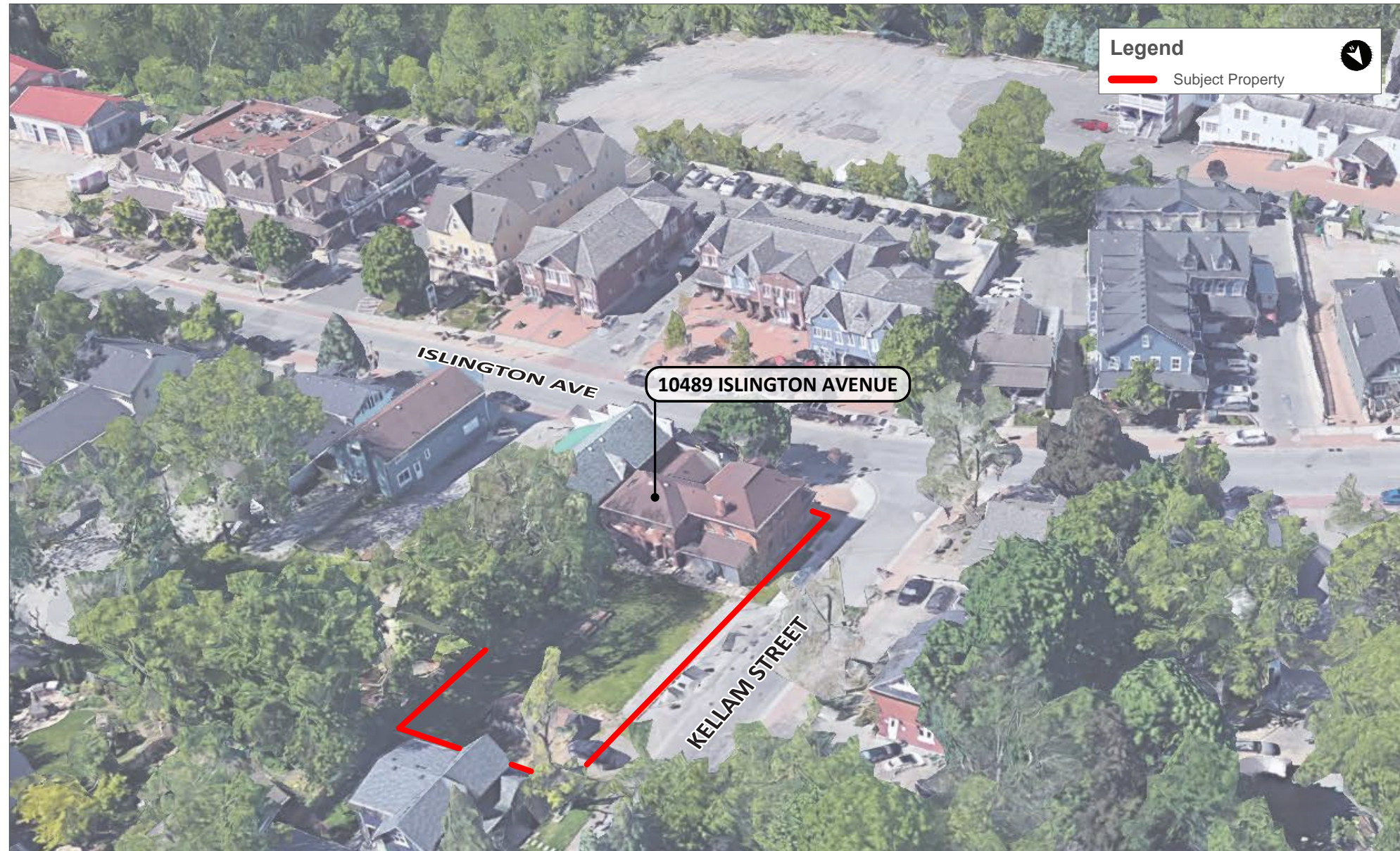
Aerial Photograph of Subject Property - Prepared by Weston Consulting
