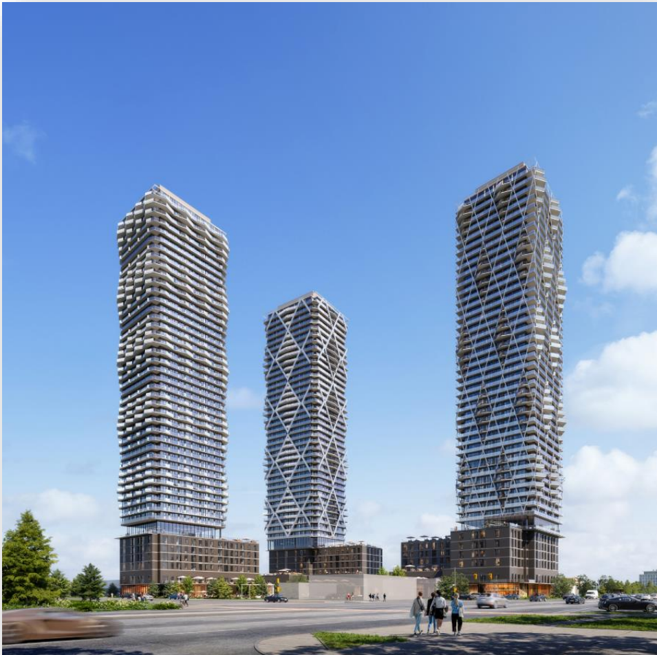
South East Façade View Looking North West
