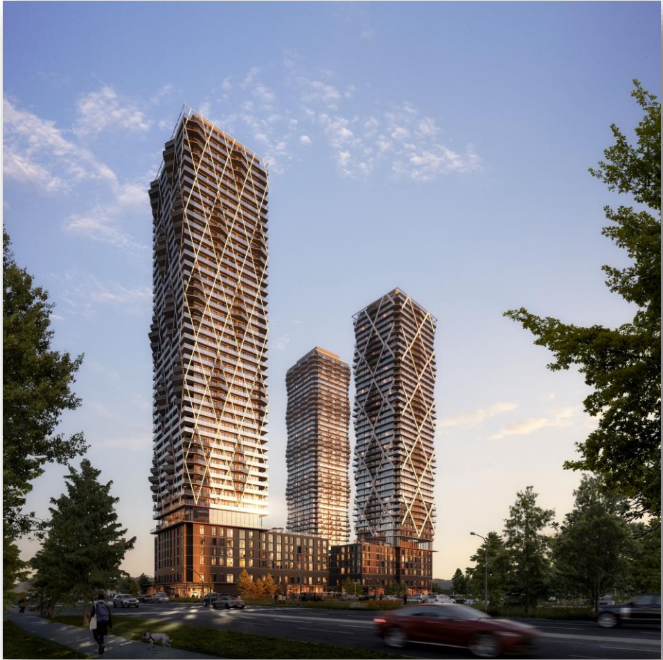
North Façade View Looking South West
