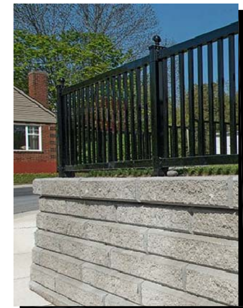
SIENNA STONE RETAINING WALL & GUARDRAIL (BROCHURE PHOTO)
