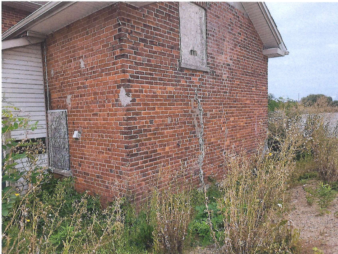
Photo 2 - View of East side showing large vertical cracks between foundation and window
