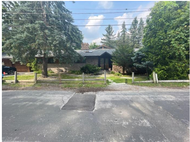
Photo 23 Modernist residence, 18 Mill Street, looking north
