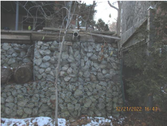
Base of Tree 5 with gabion basket supported patio to south
