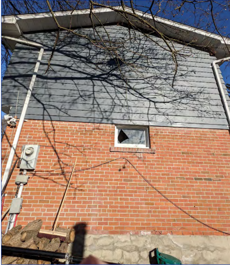
Photo 14: View of the south elevation
