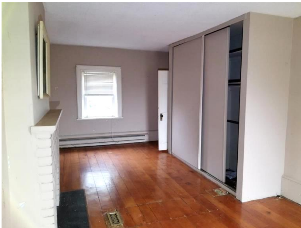
Figure 37: North room on the second storey. A closet was added when the function of the room changed.
