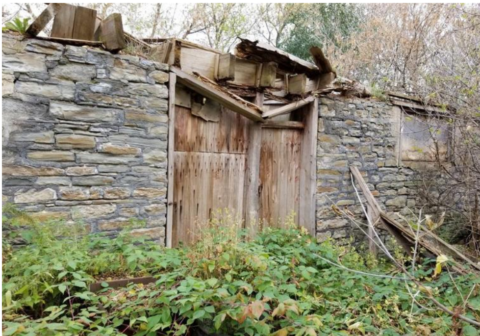
Figure 61: West façade and doors of the stone barn foundation.
