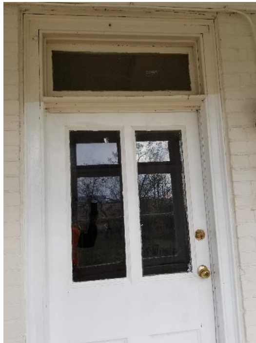
Figure 26: Front door on the west façade of the Main Block.
