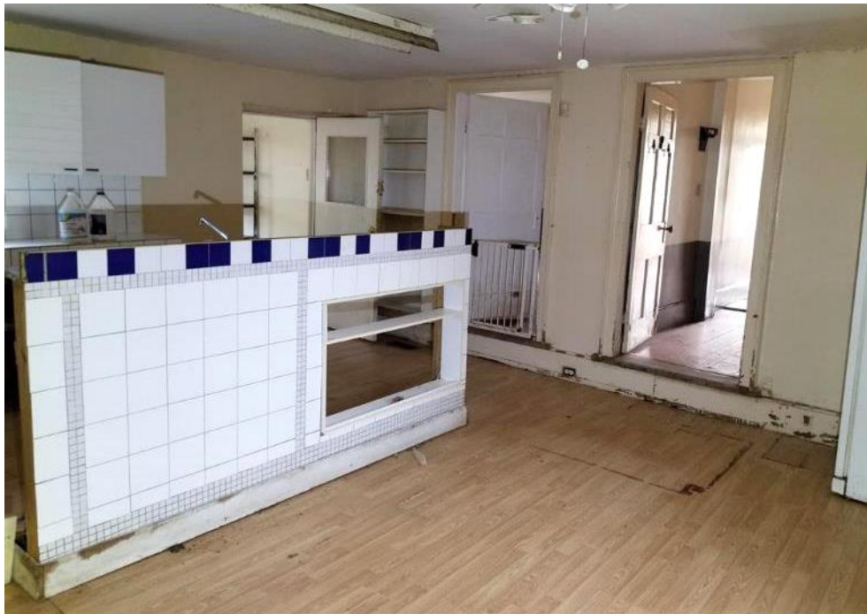
Figure 51: Interior of the East Wing facing west. Doorways to the Main Block to the west and South Addition to the south.
