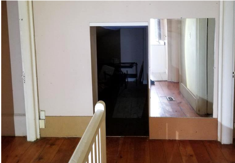
Figure 53: Entrance to the second storey of the East Wing, from the Main Block.
