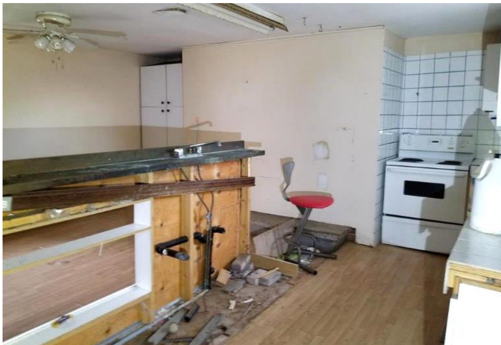
Figure 52: Interior of the East wing facing the east wall. Covered hearth in the centre of the wall.
