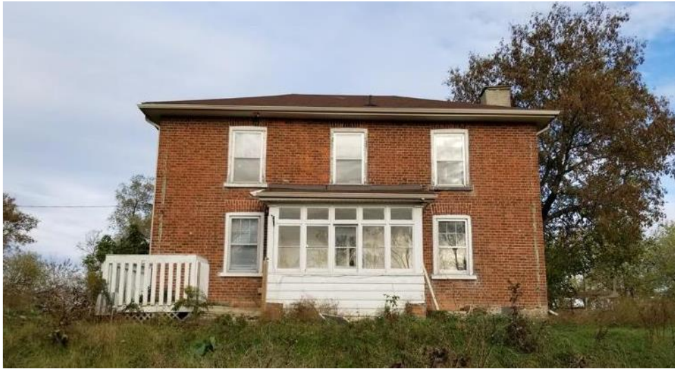
Figure 16: West façade of John Fleming House.
