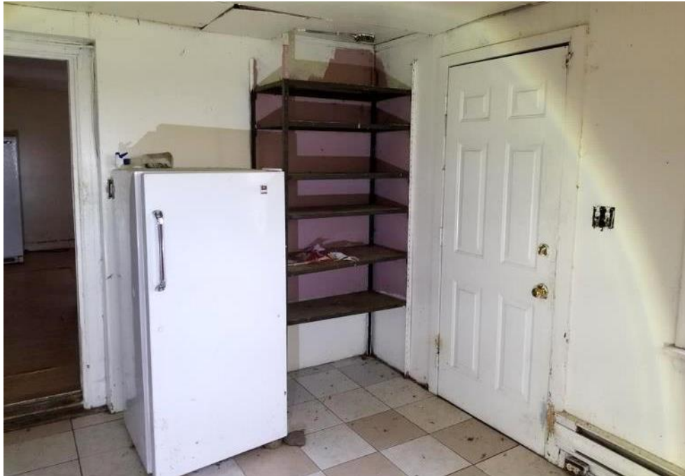
Figure 57: Facing northeast inside the South Addition with the exterior door on the east wall.
