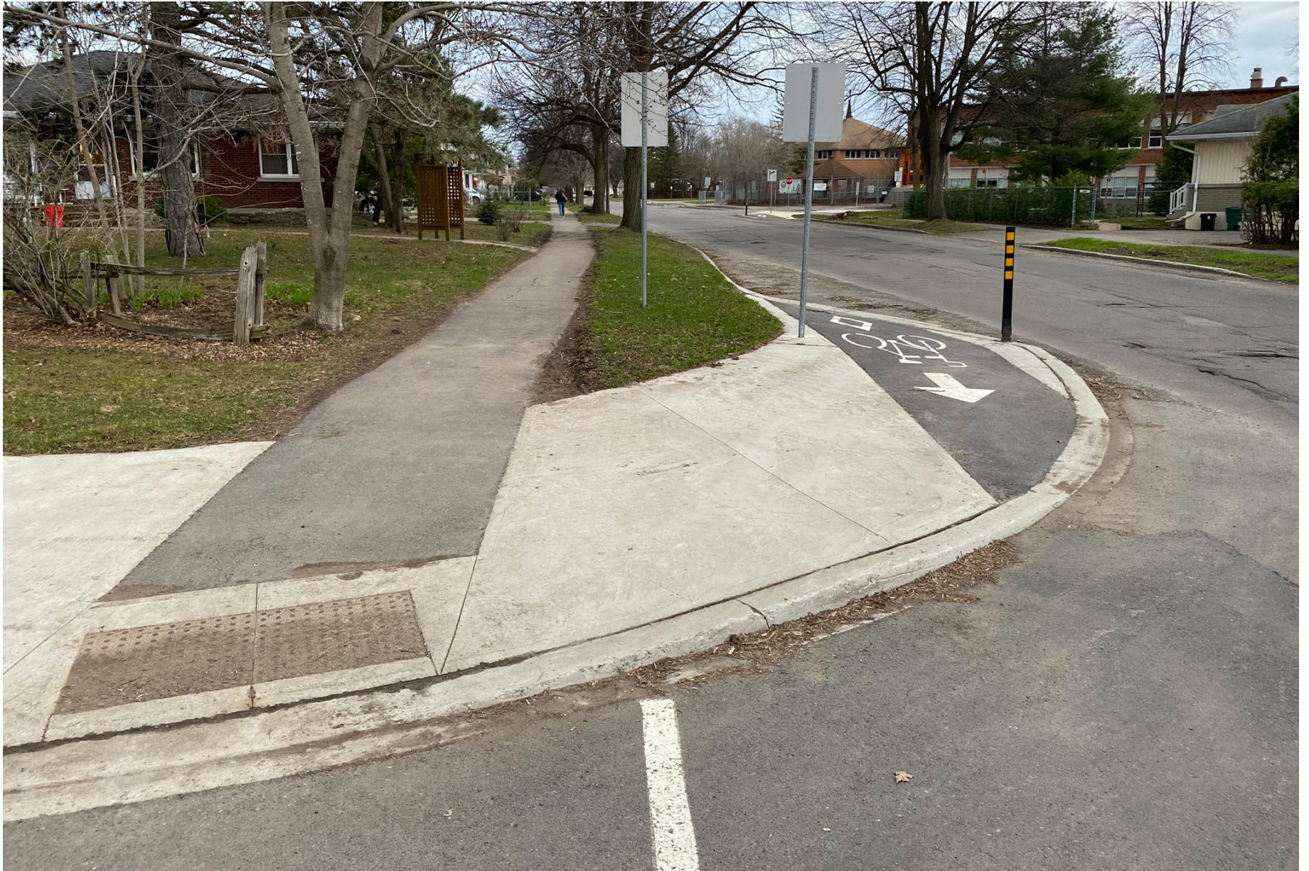
Figure 12: Chicane with Cycle Track
