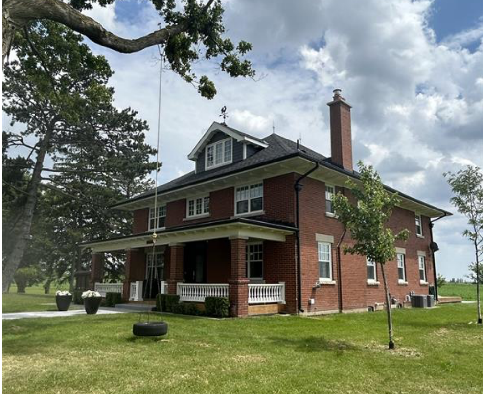
2601 King-Vaughan Road (photo taken July 2024)
