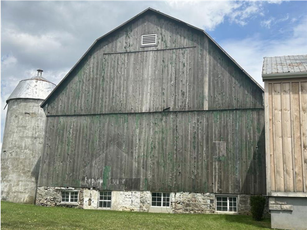
2601 King-Vaughan Road (photo taken July 2024)
