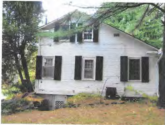
Salt box shape is evident here.
