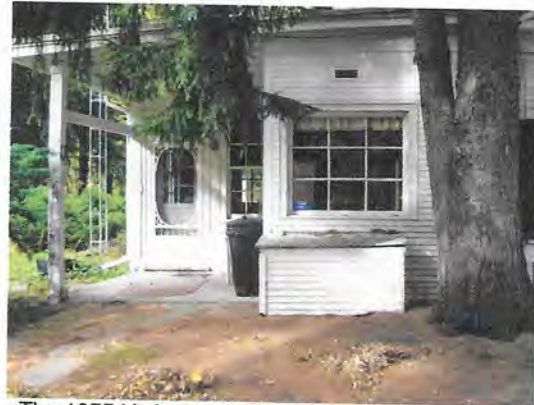
The 1955 kitchen extension, with 1910 open porch to the left
