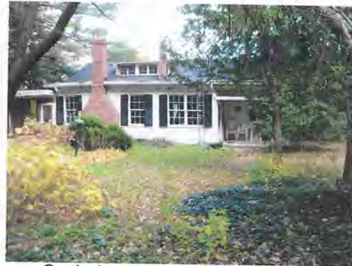
South elevation showing later additions
