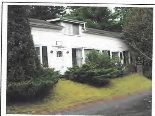
The north elevation
