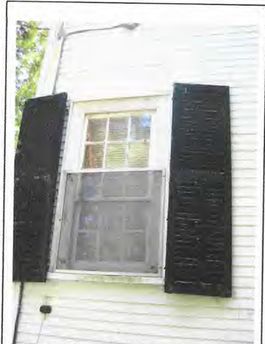
Original 9 over 6 window, west elevation
