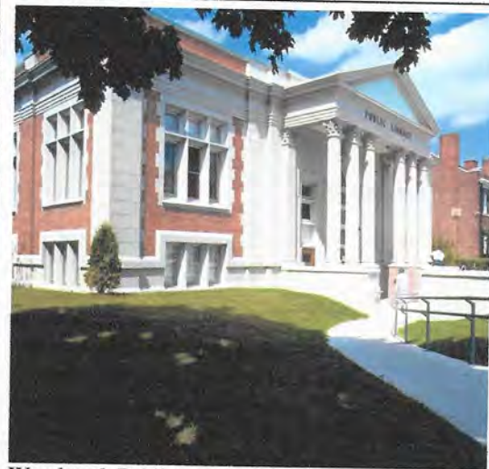
Woodstock Public Library $2.5M Renovations & Additions 1996
