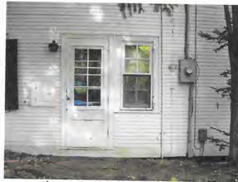
4 over 4 window, east elevation
