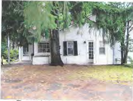
The east façade, seen through the trees
