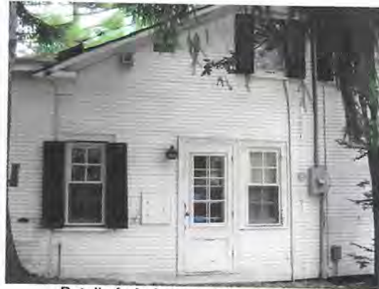
Detail of windows and door, east side
