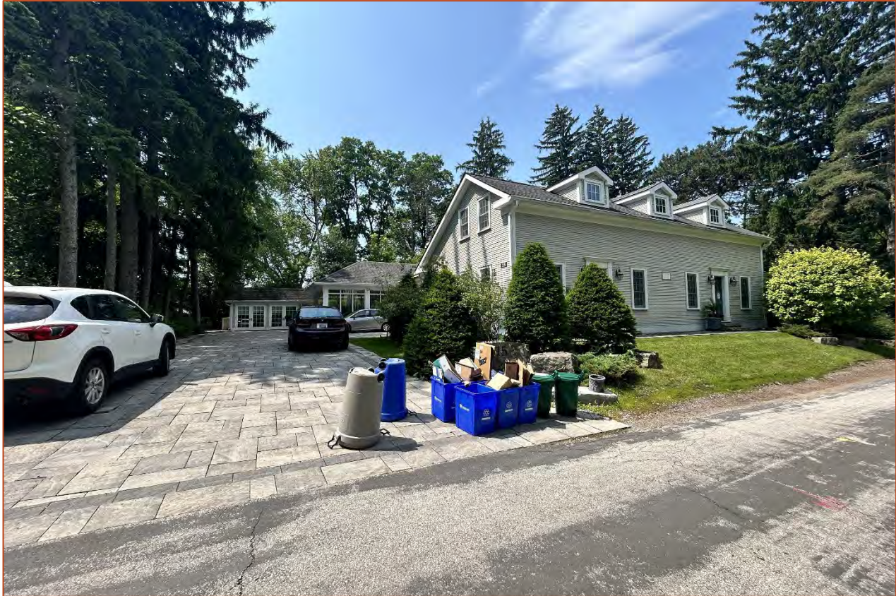
Figure 2. View southwest showing the Property
