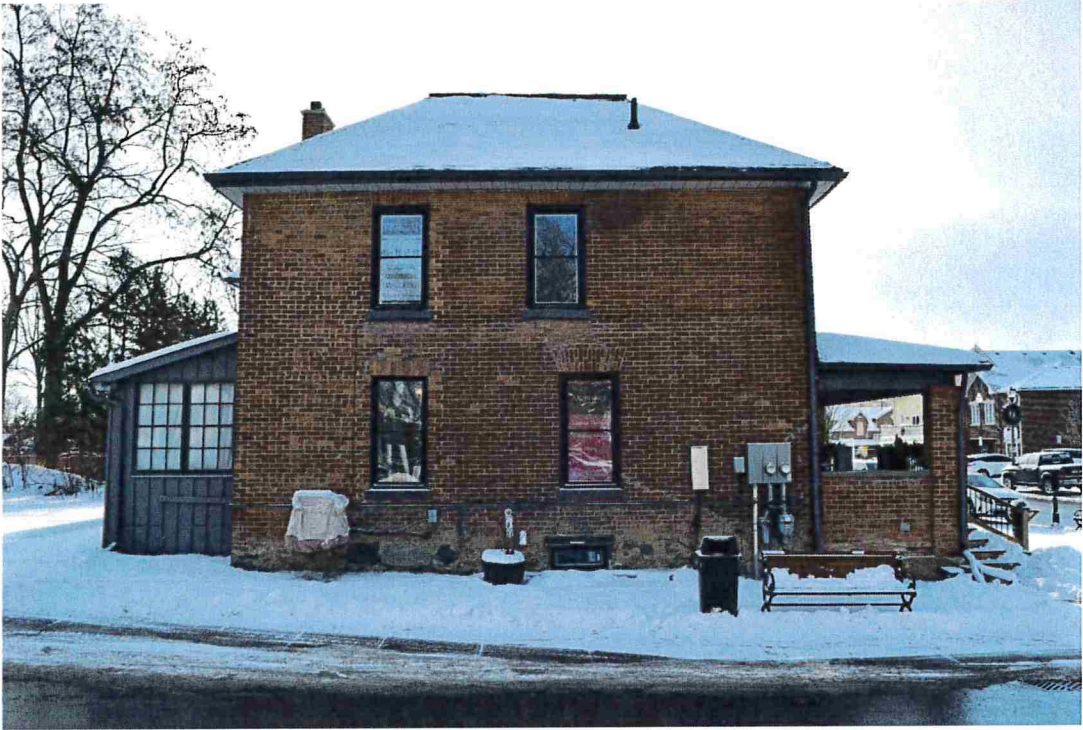
Figure 6: North façade (December 2016).
