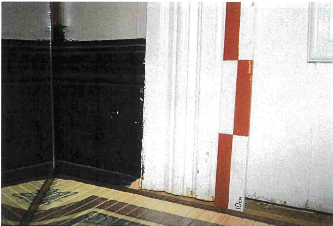
Figure 18: Original baseboard and door architraves (December 2016).
