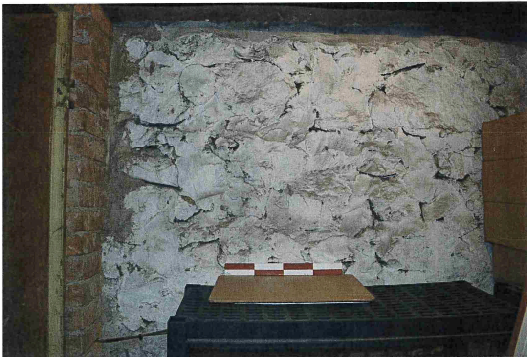
Figure 9: Rubble foundation masonry as seen from the basement (December 2016).
