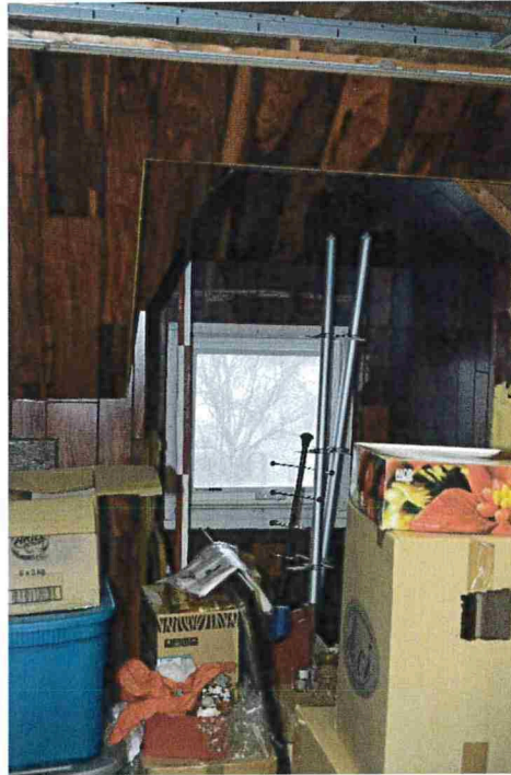
Figure 24: Interior of the attic, facing the dormer (December 2016).
