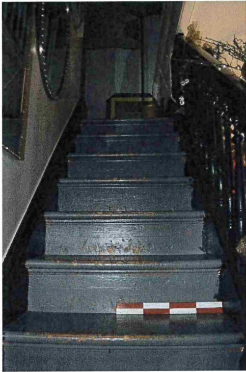
Figure 19: The stairs to the second level (December 2016).
