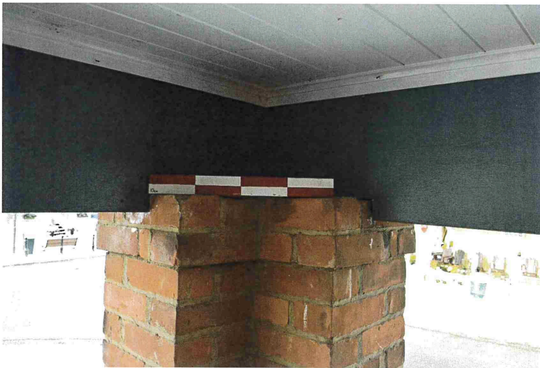
Figure 15: Brick pier, fascia, and ceiling (December 2016).
