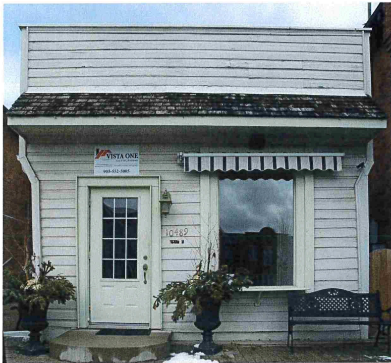
Figure 10: West façade of the Ice Cream Shop.
