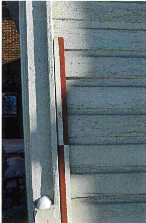
Figure 15: Detail of the front façade corner board and shiplap cladding.
