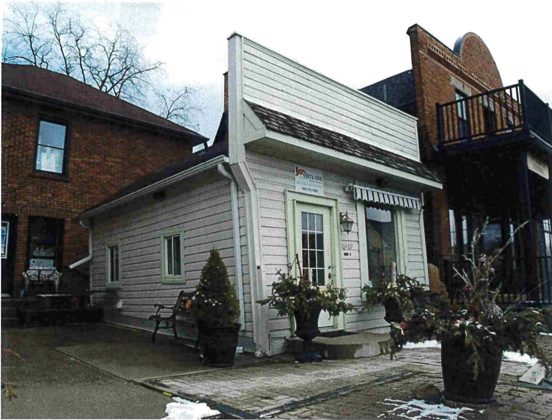
Figure 11: North sidewall and west façade.
