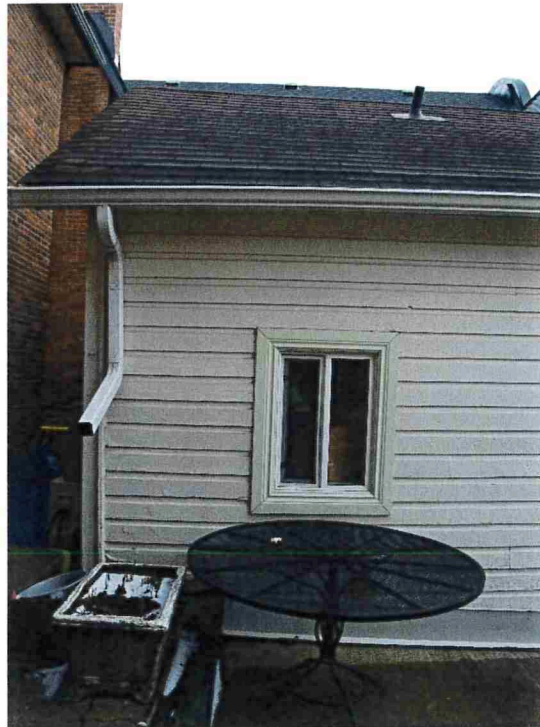
Figure 17: East window on the north sidewall.
