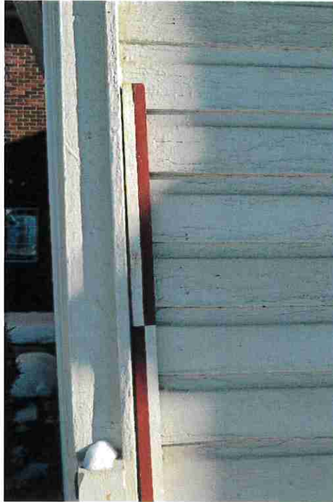
Figure 48: Detail of the corner board and shiplap cladding.
