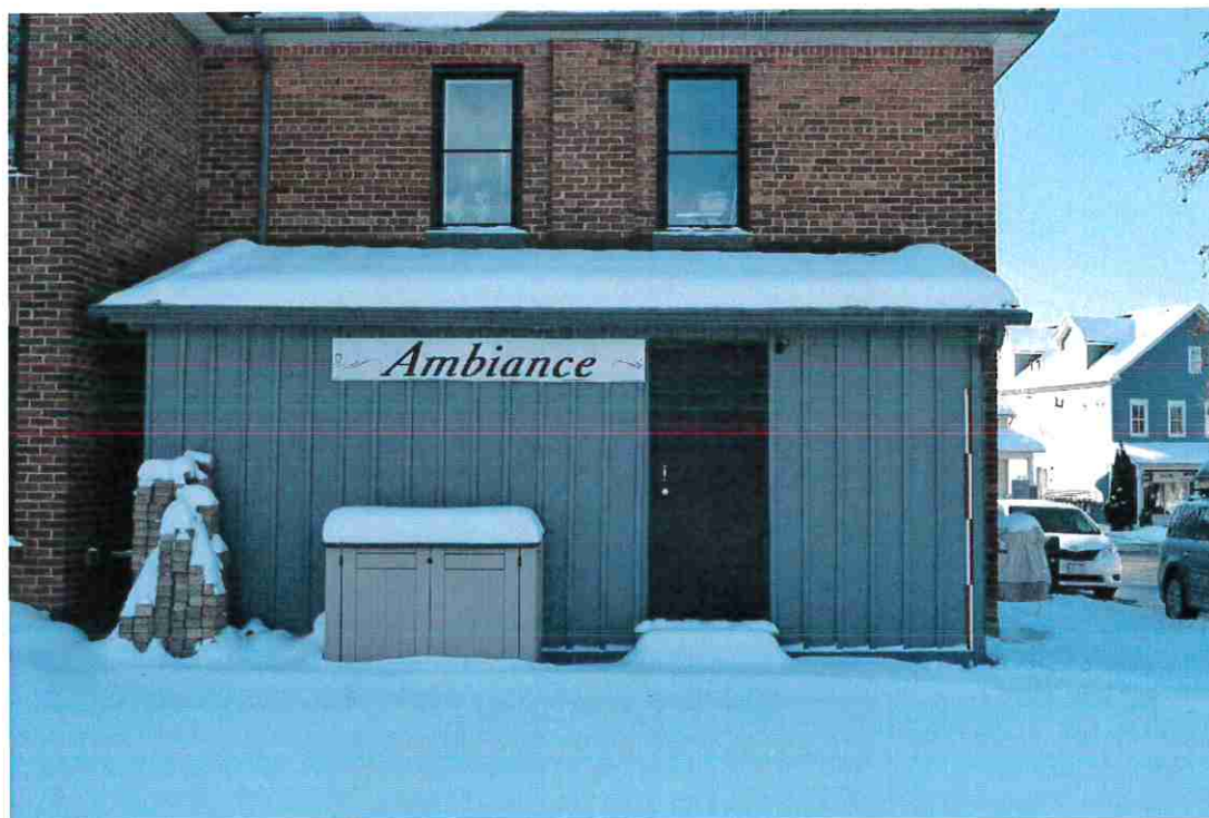
Figure 30: East façade of the wood frame addition.
