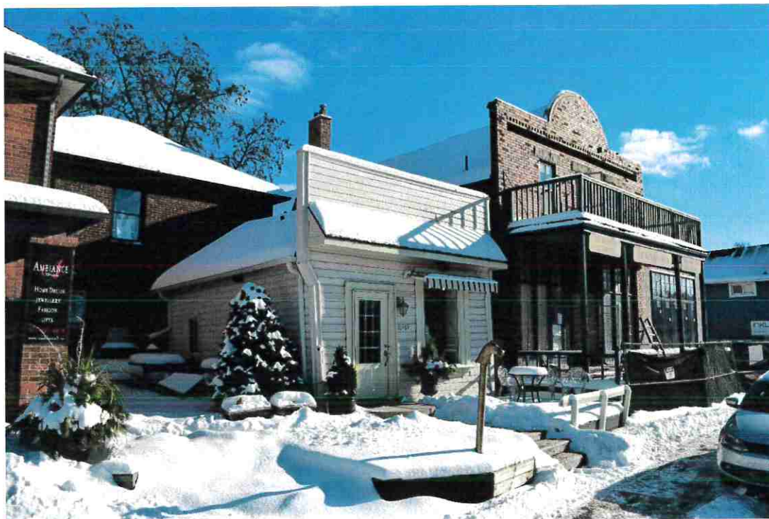
Figure 46: North and west façades of the shop.
