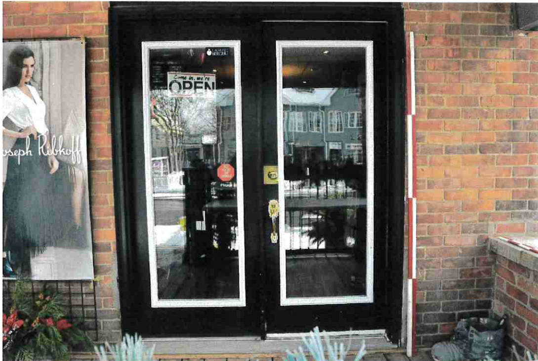
Figure 27: South doors on the west façade.
