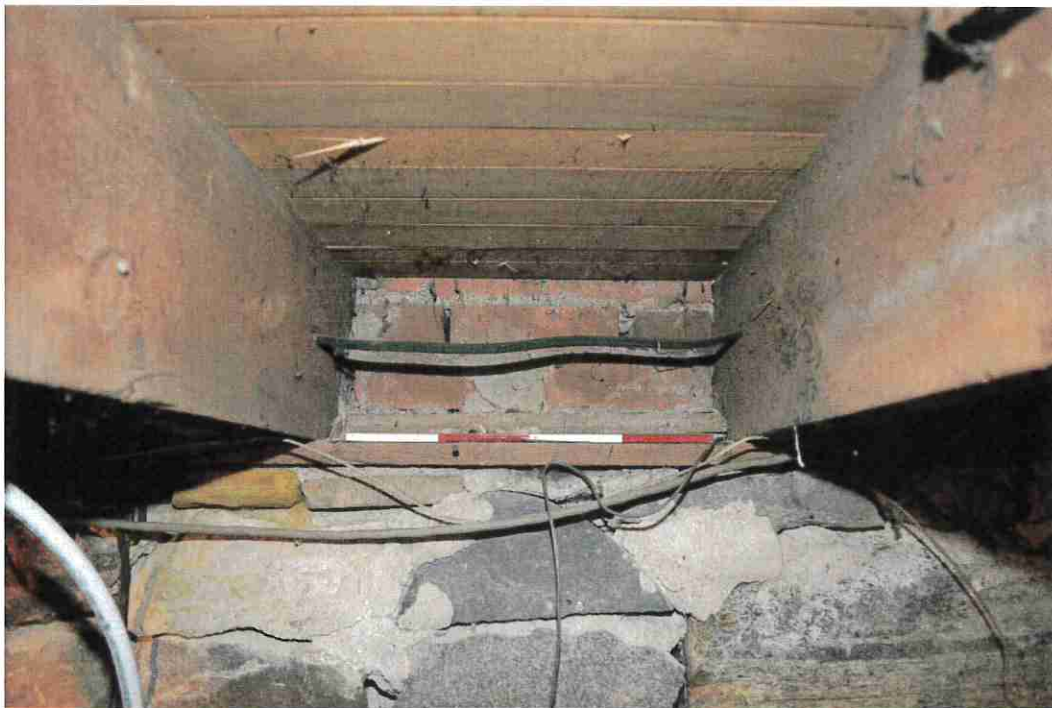
Figure 38: Joists and floorboards in the main block basement.
