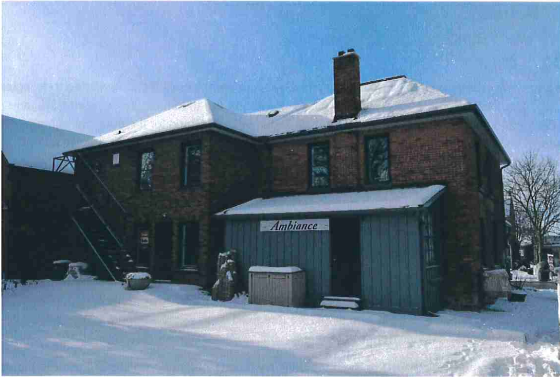
Figure 17: East and north façades of the house.
