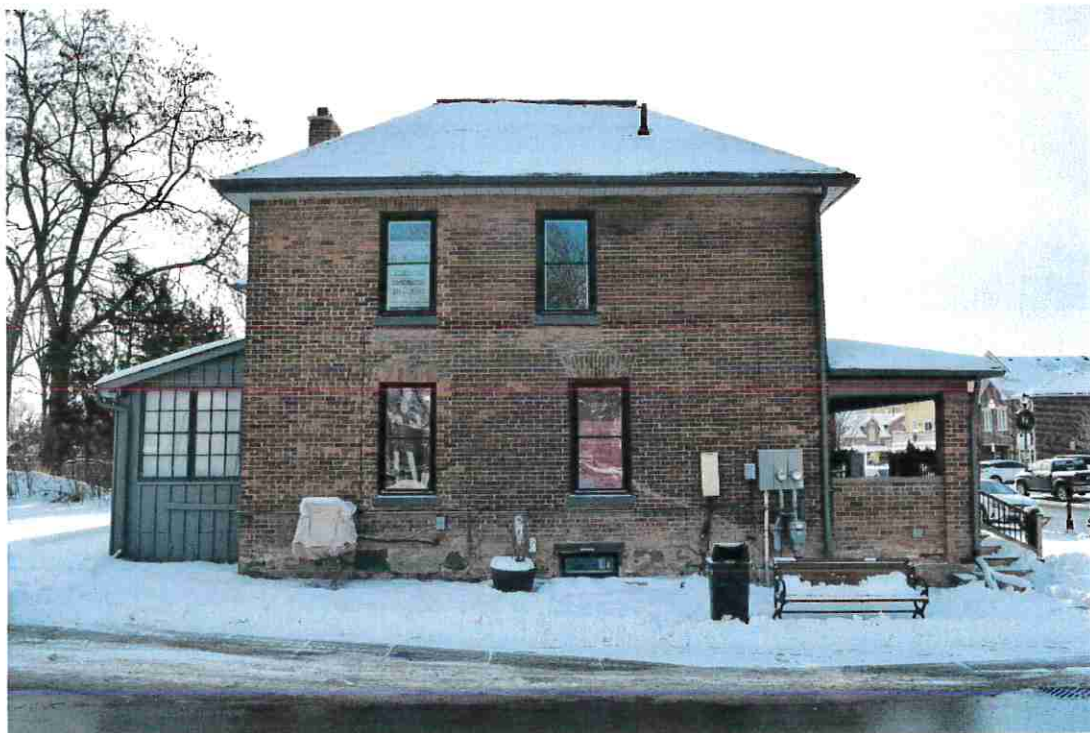
Figure 16: North façade of the house.
