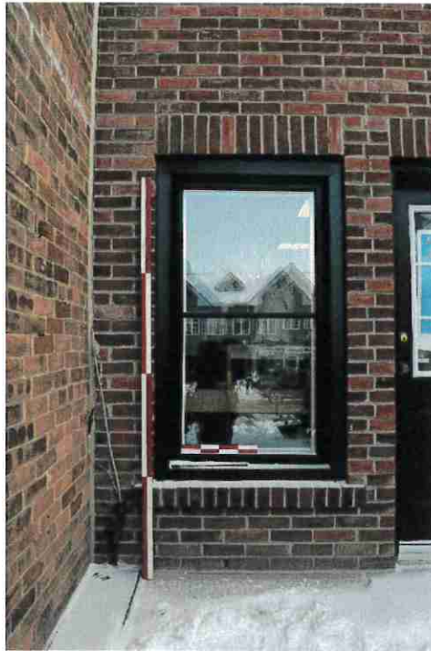
Figure 42: Typical window of the brick wing.
