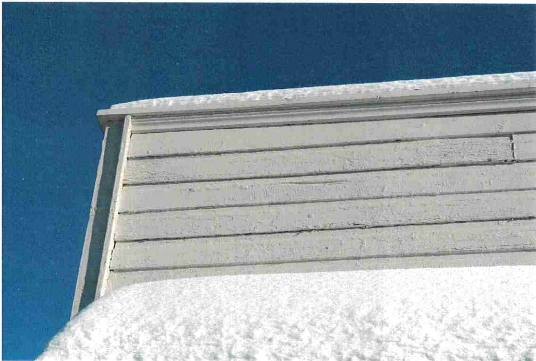
Figure 49: Cornice at the parapet on the west façade.
