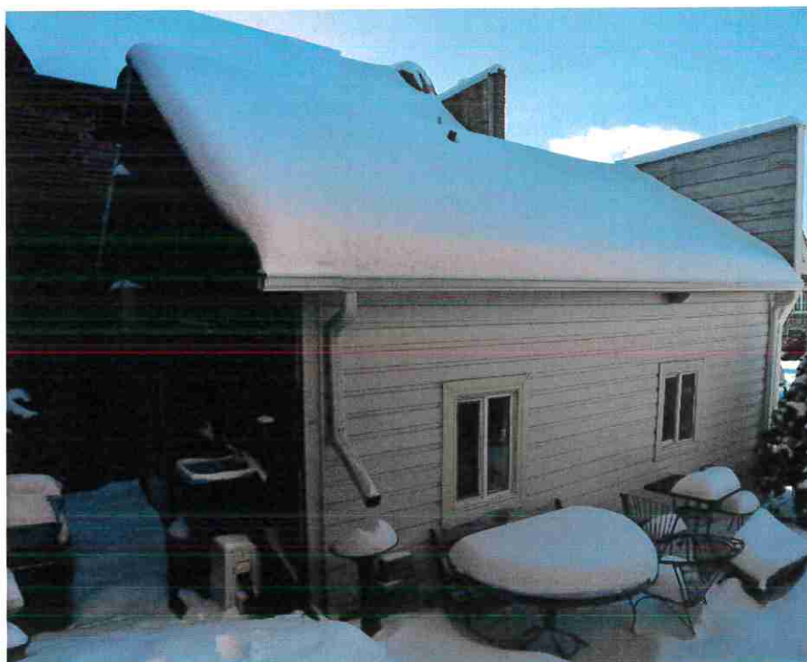
Figure 47: East and north façades.
