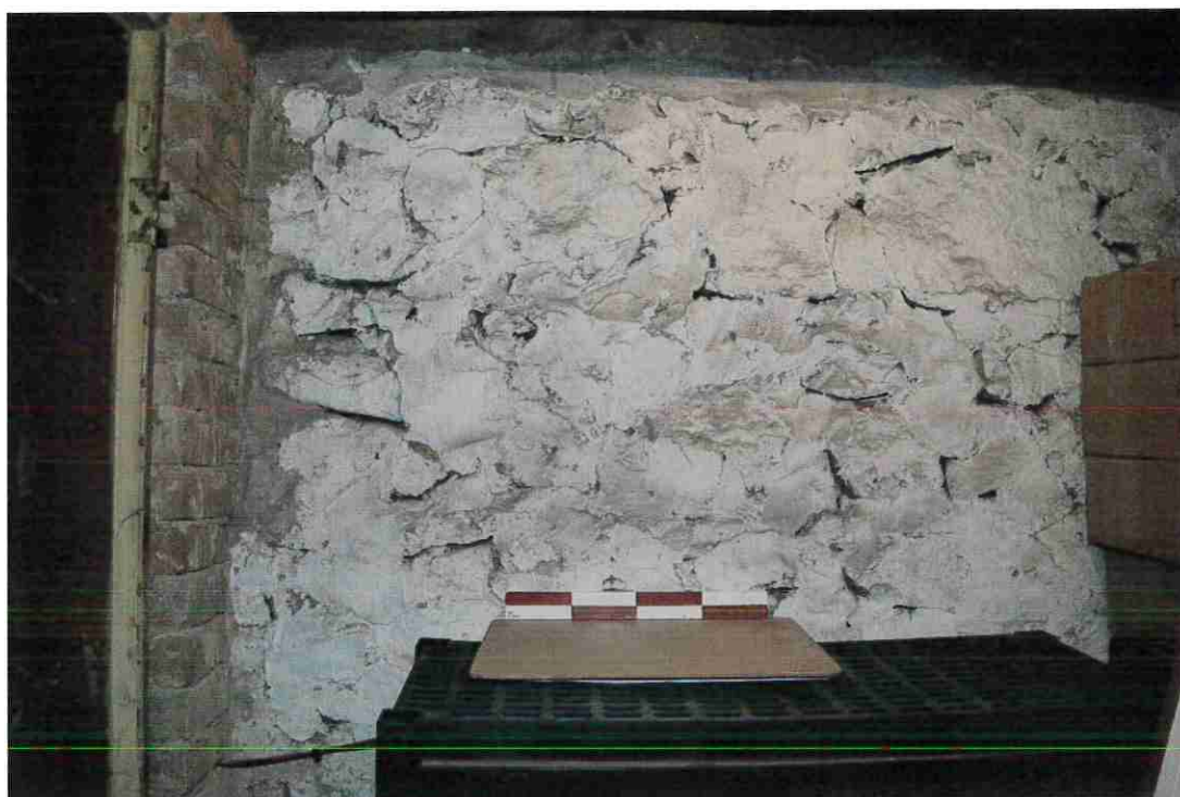
Figure 21: Rubble foundation masonry as seen from the basement.
