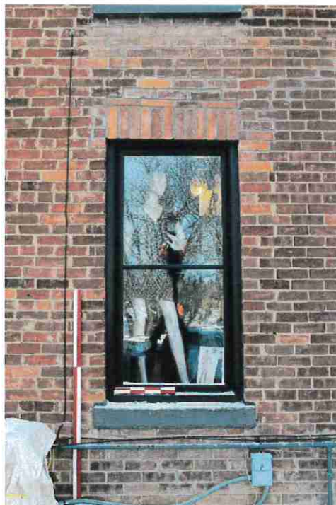
Figure 24: Window in the east extension.
