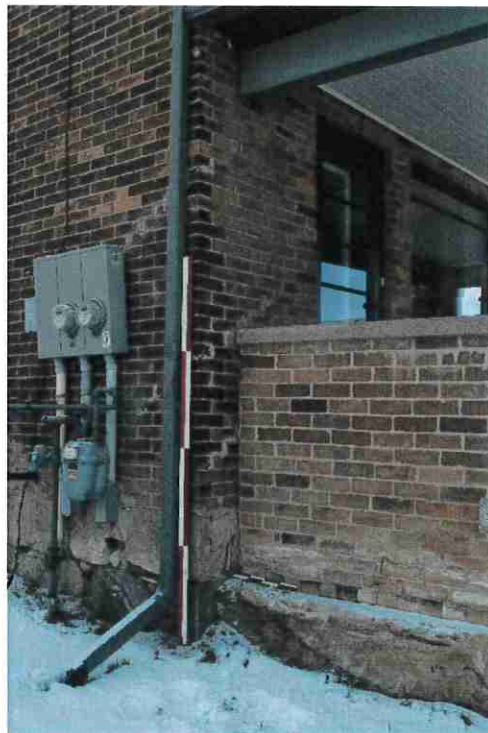
Figure 28: Connection between the verandah and main block.
