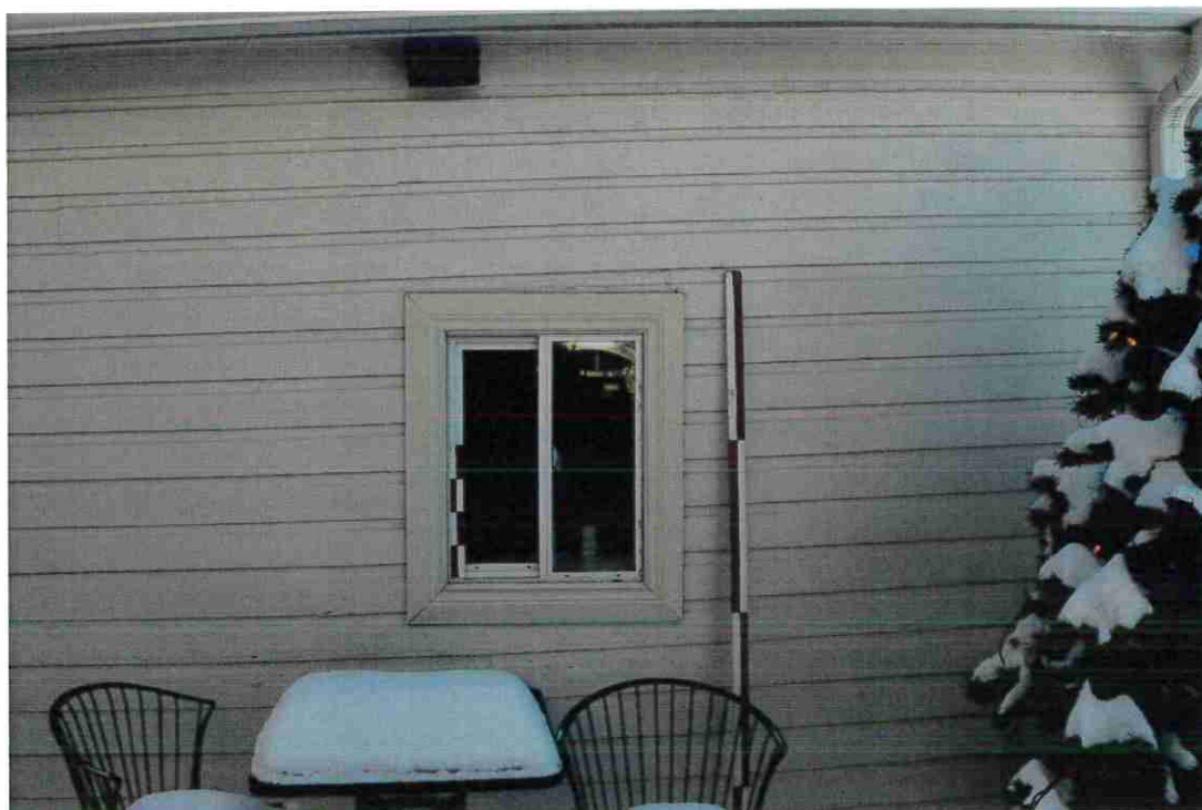
Figure 50: Window on the north wall.
