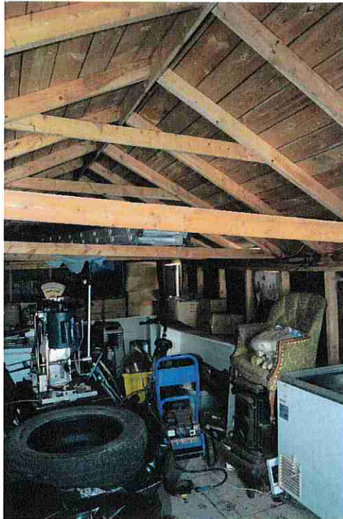
Figure 59: Dimensional lumber roof trusses in the garage.
