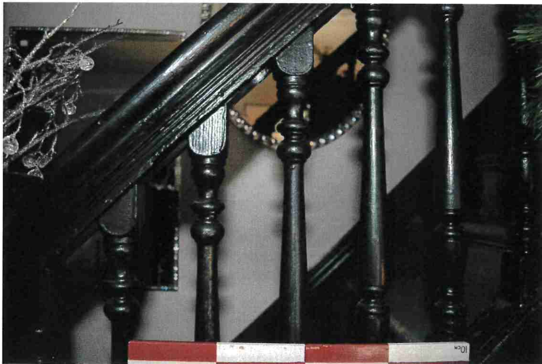
Figure 35: Balustrade of the stairs to the second level.
