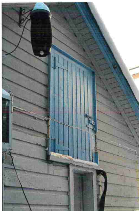
Figure 51: Door in the east gable.
