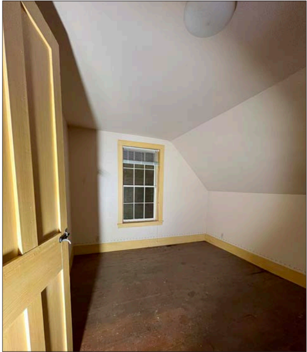
30. Munshaw house, second level, no interior work completed.
