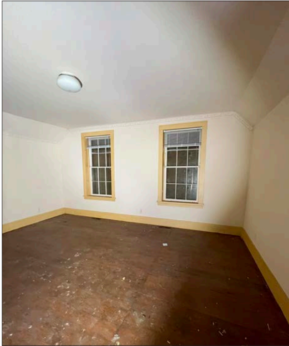
29. Munshaw house, second level, no interior work completed.
