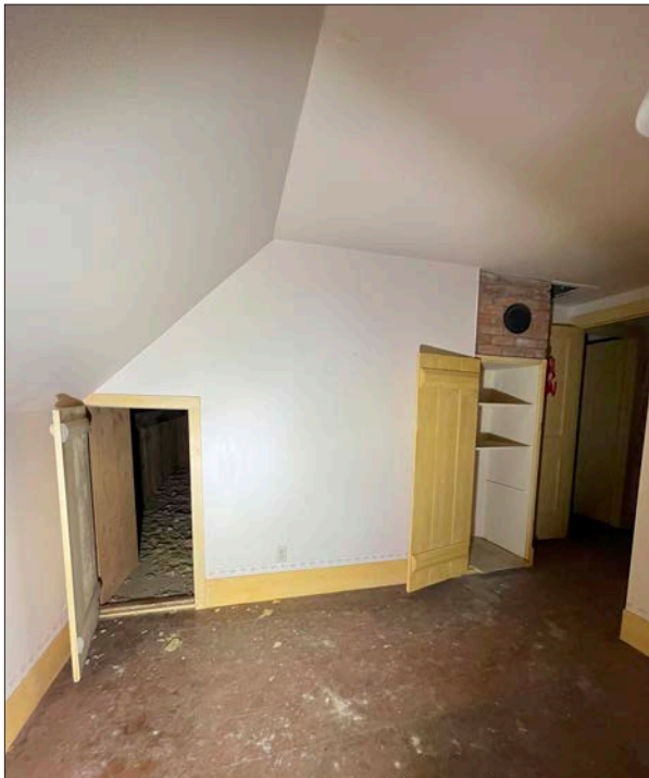
31. Munshaw house, second level, no interior work completed.
