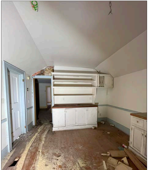
28. Munshaw house, ground level, no interior work completed.
