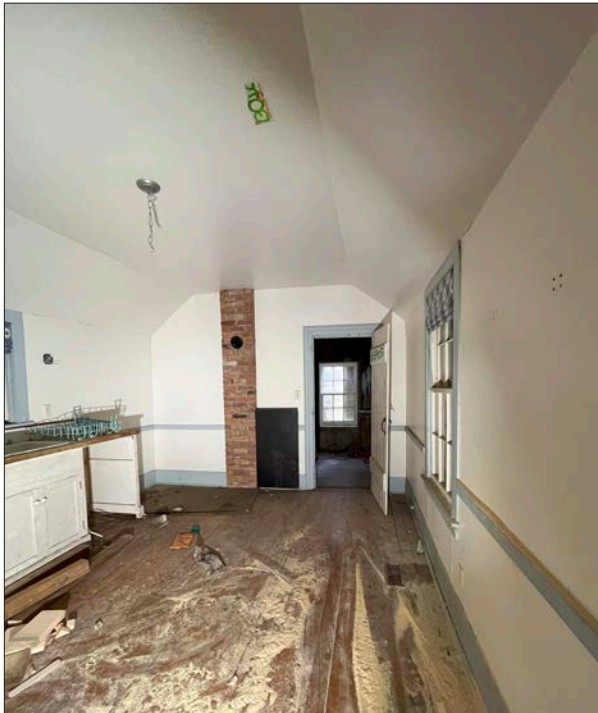
27. Munshaw house, ground level, no interior work completed.
