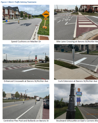
The following images show some of the traffic calming treatment installations.
