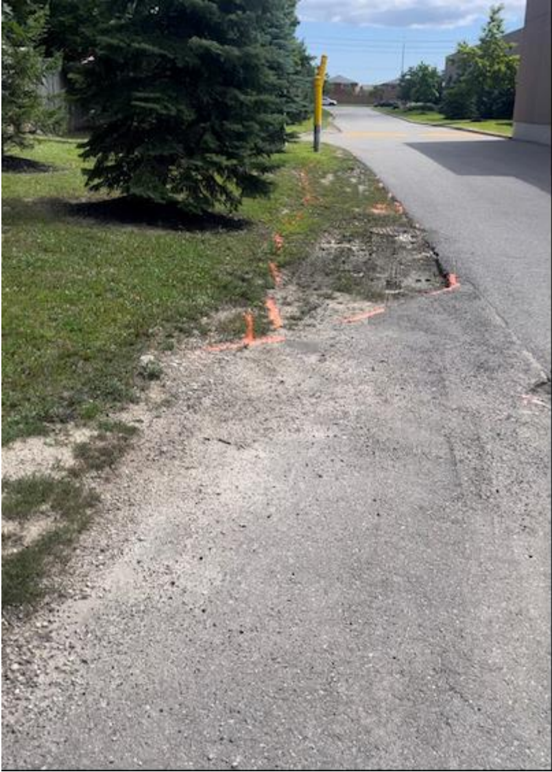
Laneway expansion markings. Facing South of the laneway towards Langstaff Ave.
