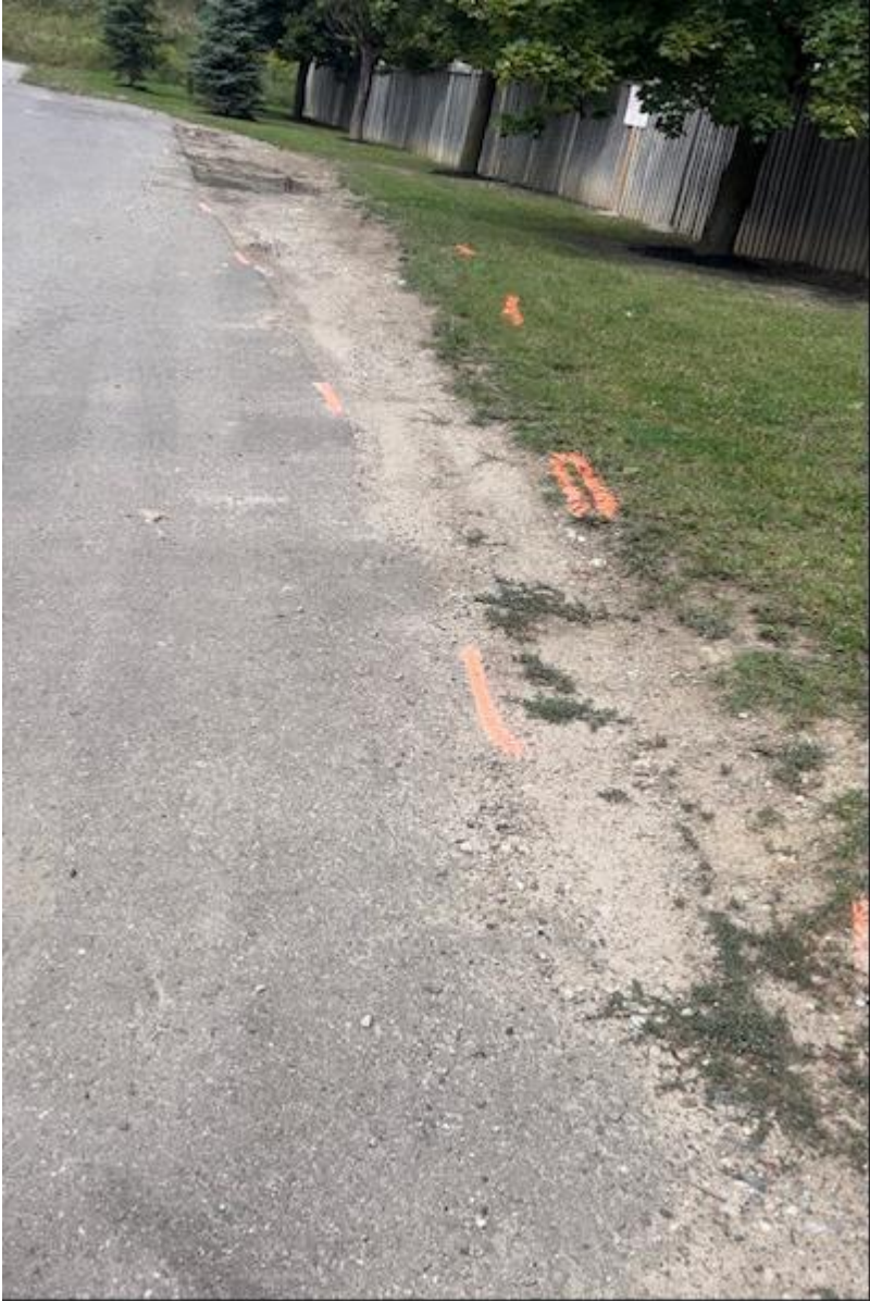
Laneway expansion markings. Facing North of the laneway.
