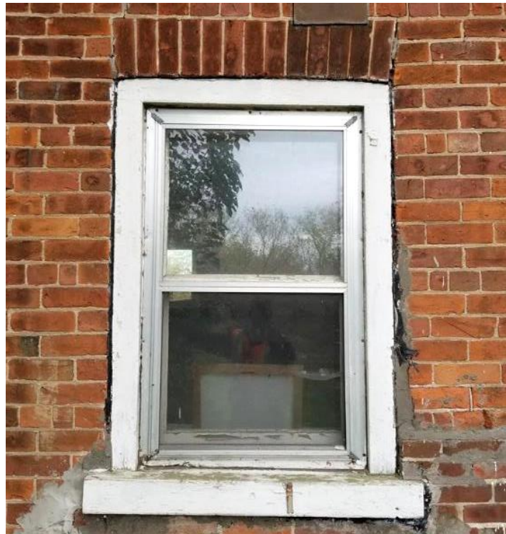
Figure 48: Typical window on the East Wing, north façade.
