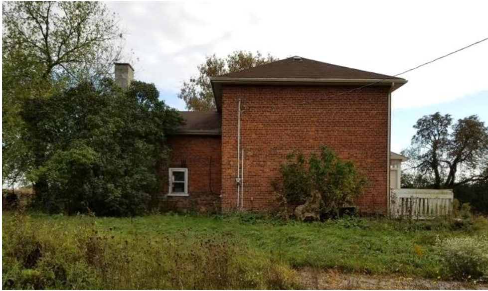
Figure 18: North façade of the Main Block and East Wing.
