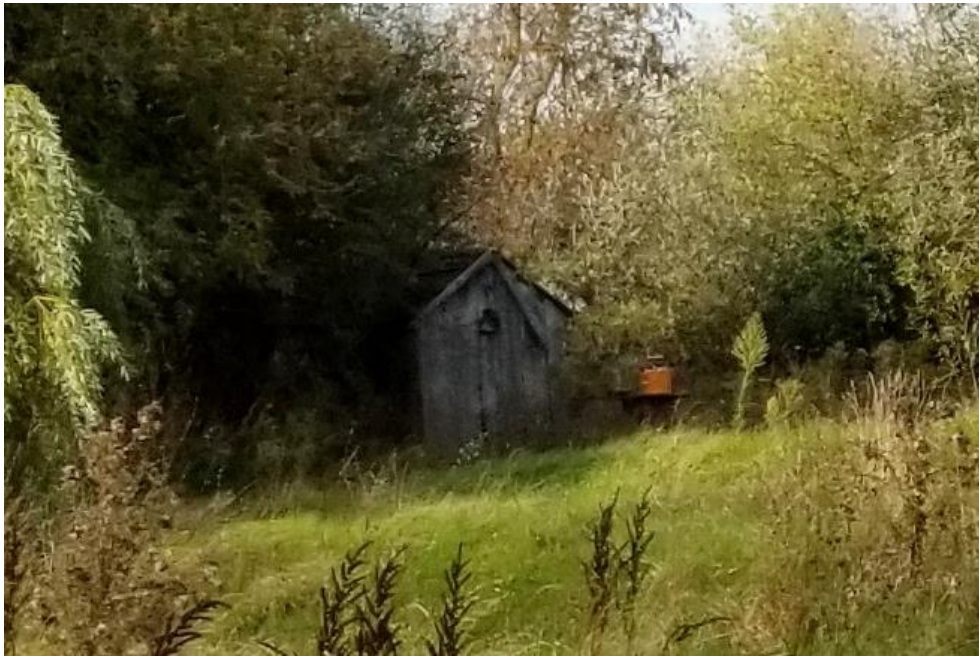
Figure 59: View of the North Outbuilding, looking north.
