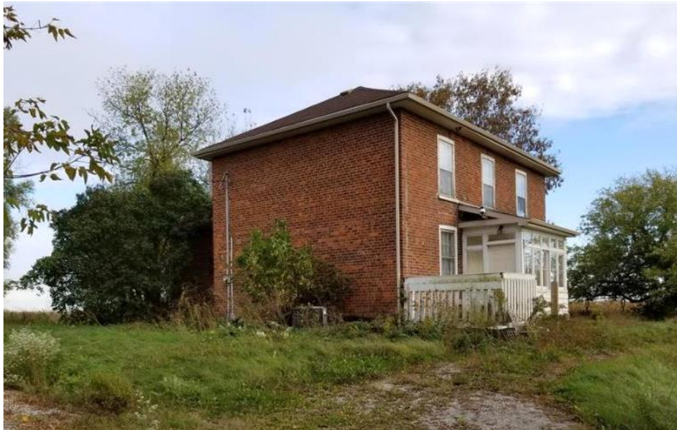
Figure 17: West and north façades.
