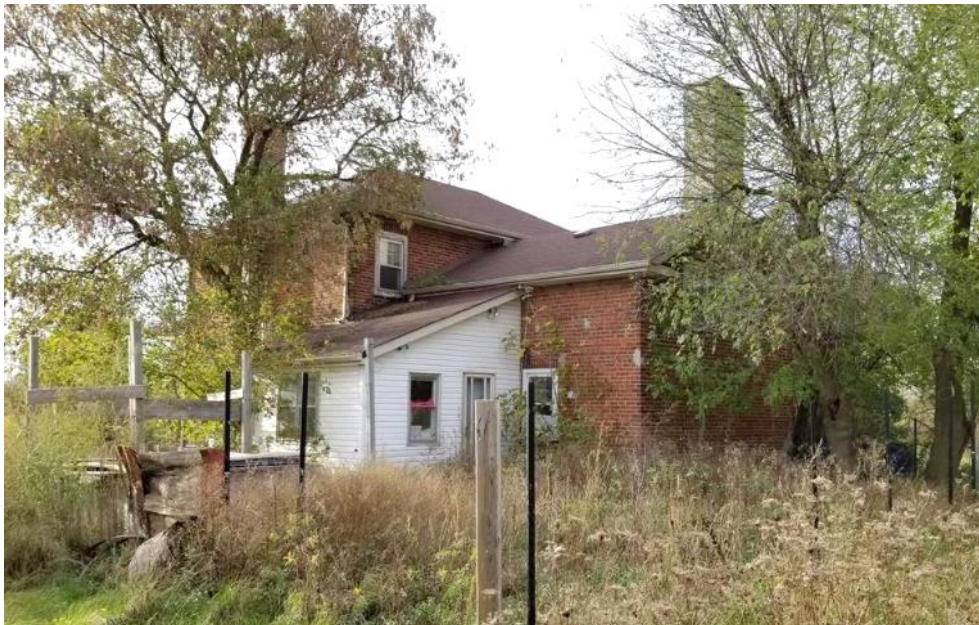
Figure 19: South and east façades.
