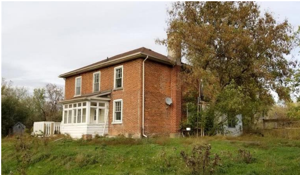
Figure 21: South and west façade.
