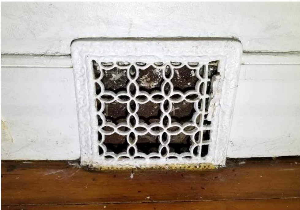
Figure 35: Decorative grate in the south wall of the northwest room.
