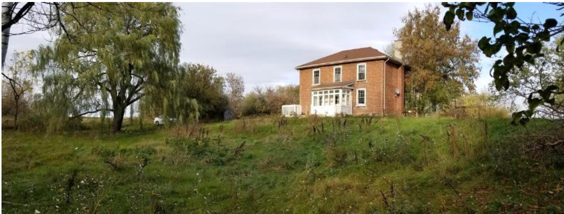
Figure 10: Facing northeast from east of the creek, showing a rise in landform with John Fleming House.
