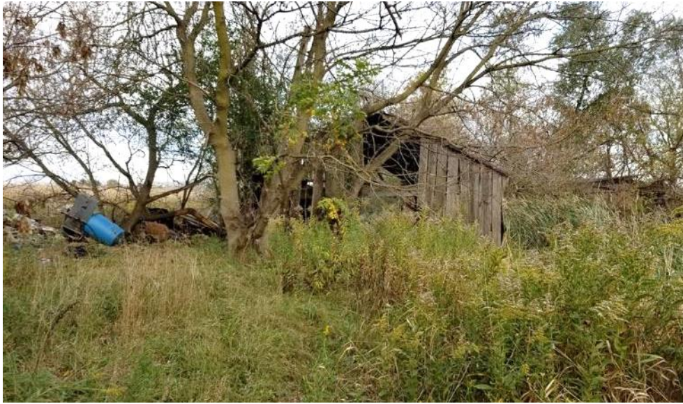
Figure 66: The west façade of the northeast outbuilding.
