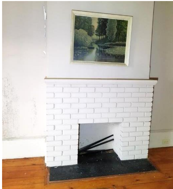
Figure 38: Relic fireplace in the north room.
