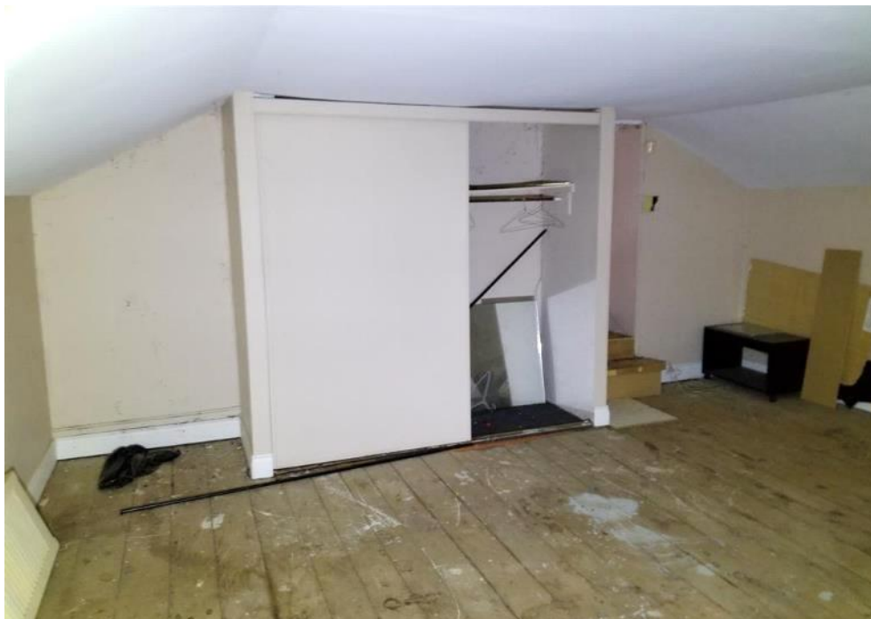
Figure 54: Second storey of the East Wing, west façade.
