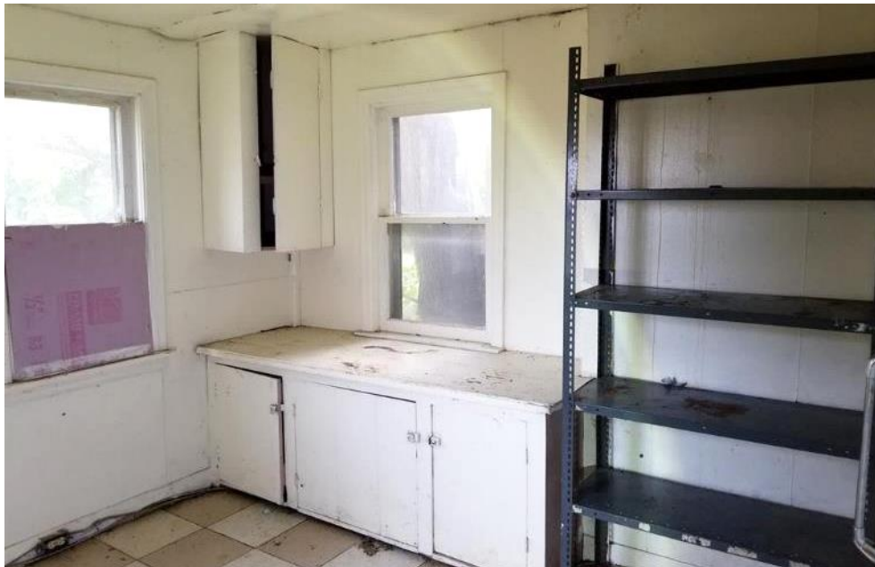
Figure 58: Facing southwest in the South Addition.
