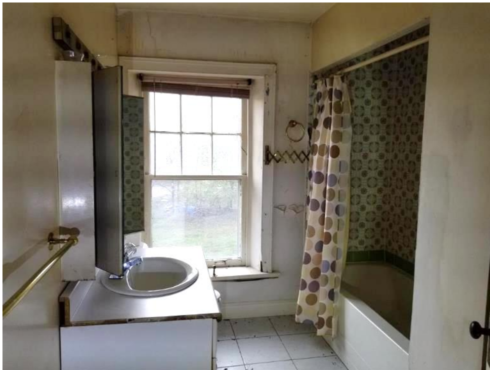
Figure 43: Bathroom at west end of the hallway.
