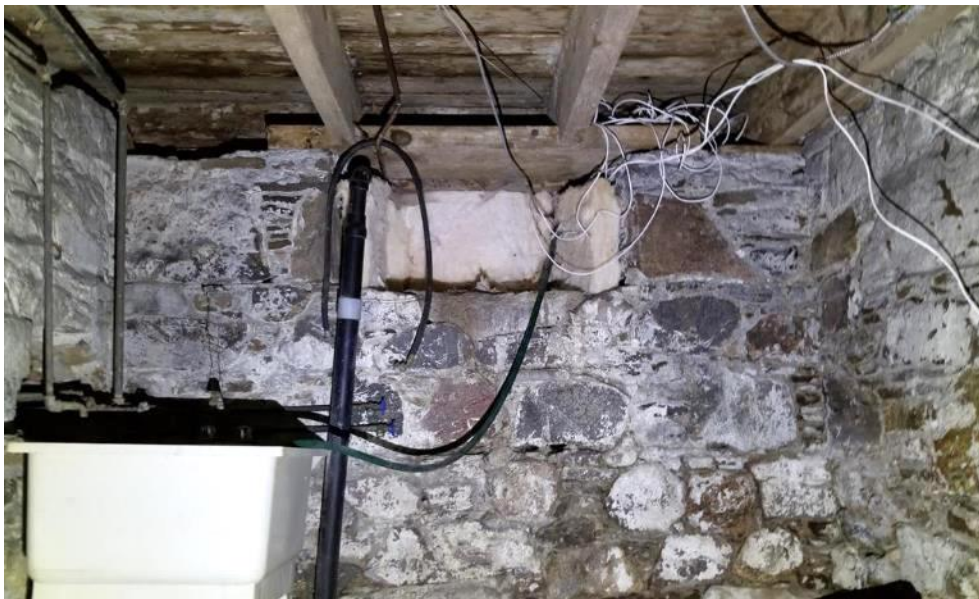
Figure 46: Basement window on south wall.
