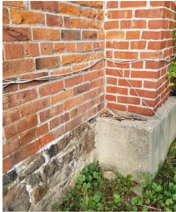
Figure 24: Chimney on the south façade of the Main Block.
