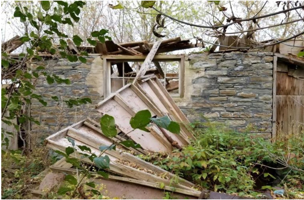
Figure 60: West façade of the stone barn foundation.
