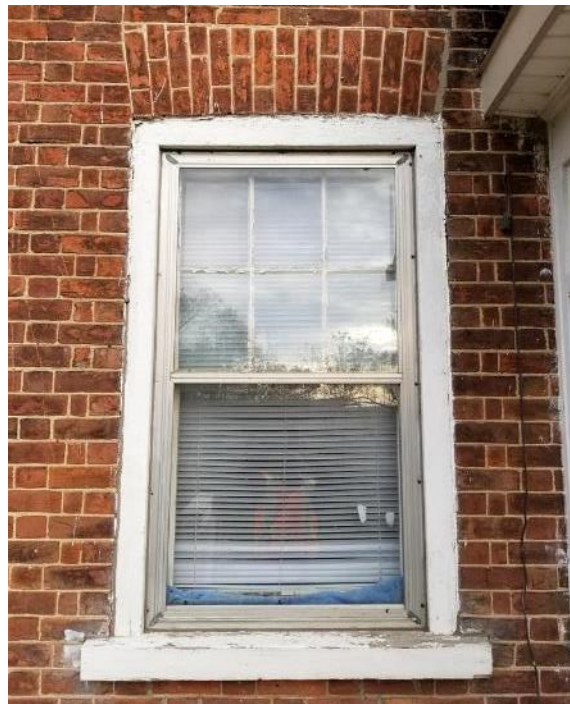
Figure 25: Typical window on the Main Block, with Flemish bond brickwork.
