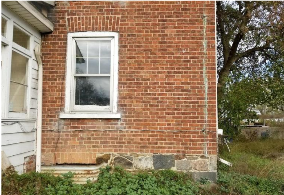
Figure 22: Detail of Flemish Bond and coursed rubble foundation on the west façade of the Main Block.
