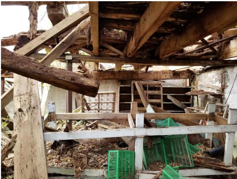
Figure 63: Interior southeast corner of the barn.
