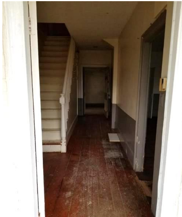
Figure 30: Central hall of Main Block.
