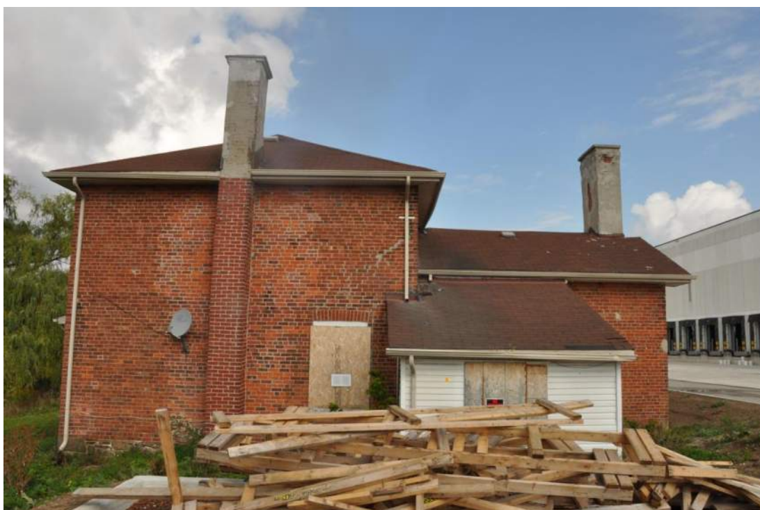
4.1.5.1.C - Existing South (Left) Elevation
