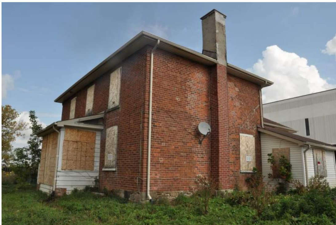
4.1.5.1.B - Existing view from southwest
