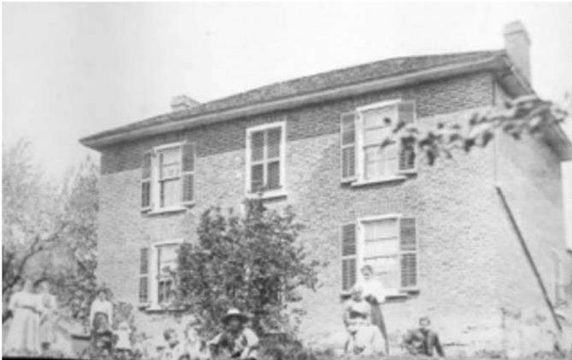
6.2.1 A – The John Fleming House in 1909 (image from the City of Vaughan Archives)
