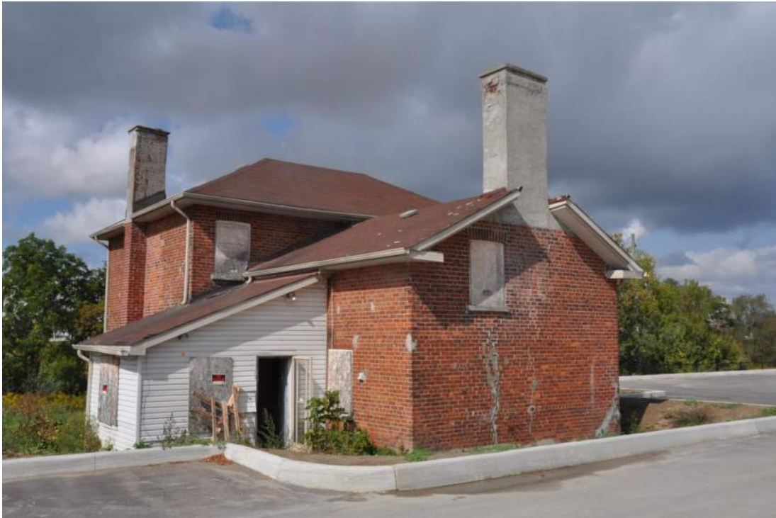
4.1.5.1.D – Existing View from Southeast
