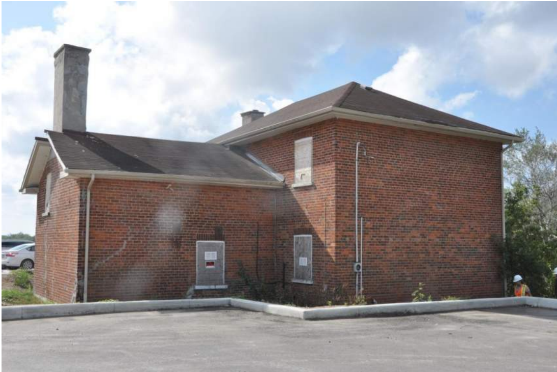
4.1.5.1.F - Existing View from Northeast
