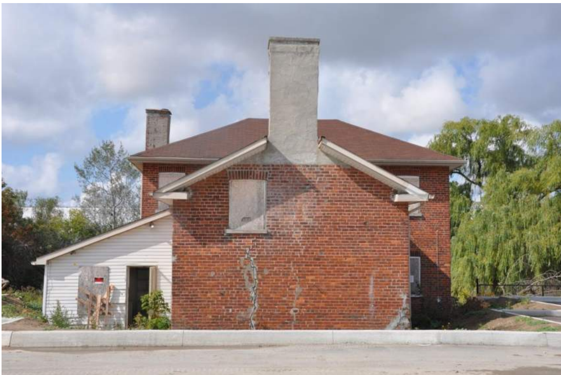
4.1.5.1.E – Existing East (Rear) Elevation
