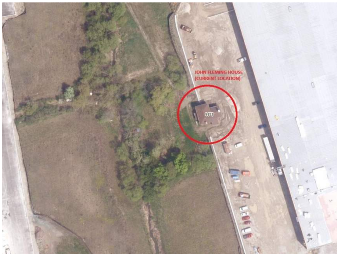
4.1.1.B - Aerial Photograph – Site Context – Enlargement
