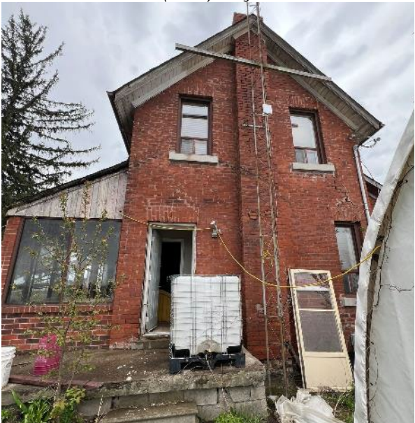
East (Rear) Façade
