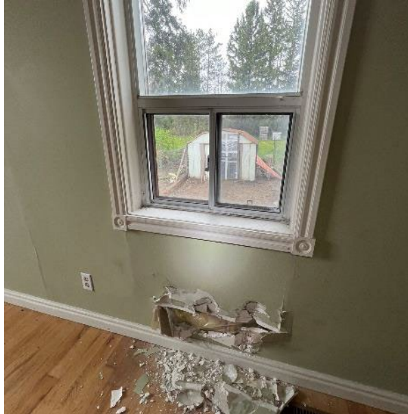
Drywall Damage
