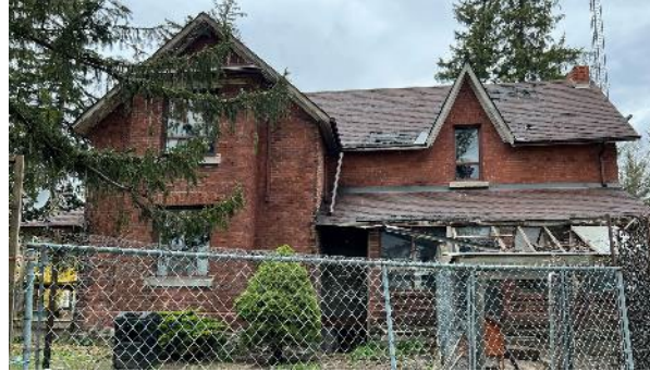
South (Side) Façade
