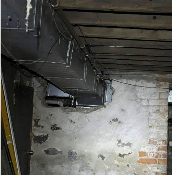
HVAC Cut through Load Bearing Wall
