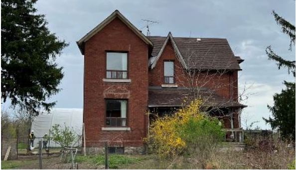
West (Front) Façade
