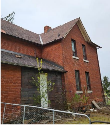
Figure 18: North Central Chimney appears to be connected to roof, second and ground floor.
