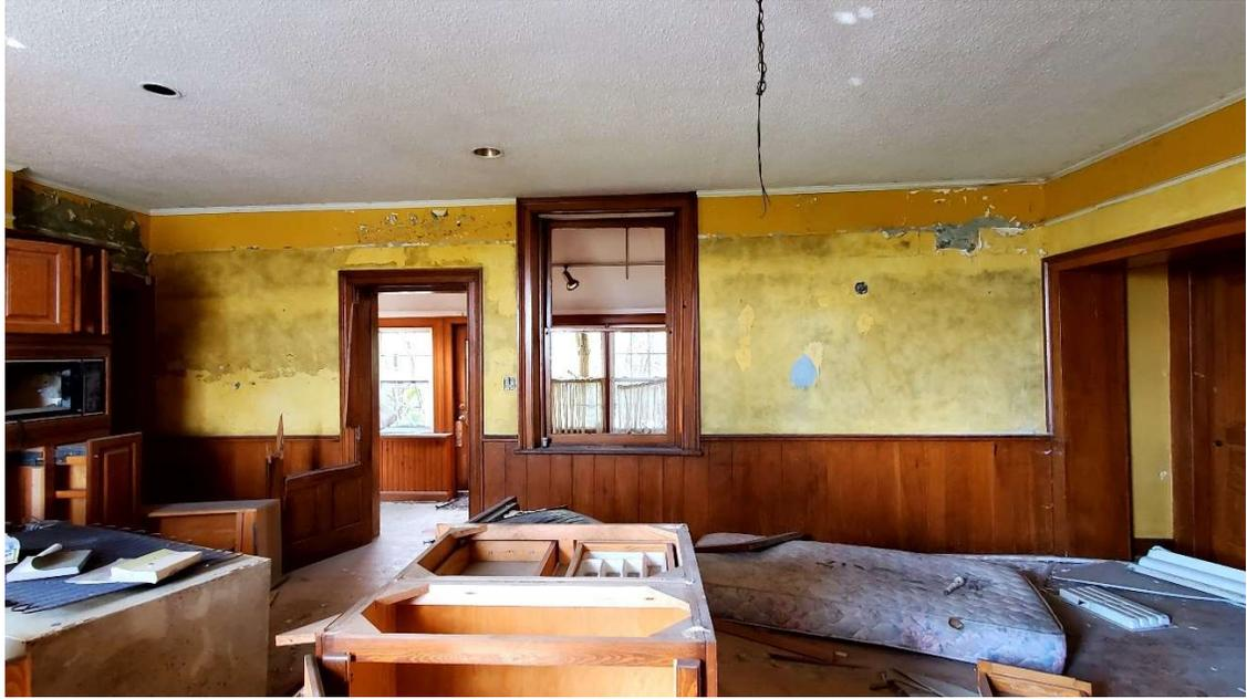
Pic. 11: Westside Wall in Kitchen; Penetration Damp-Building 1B
