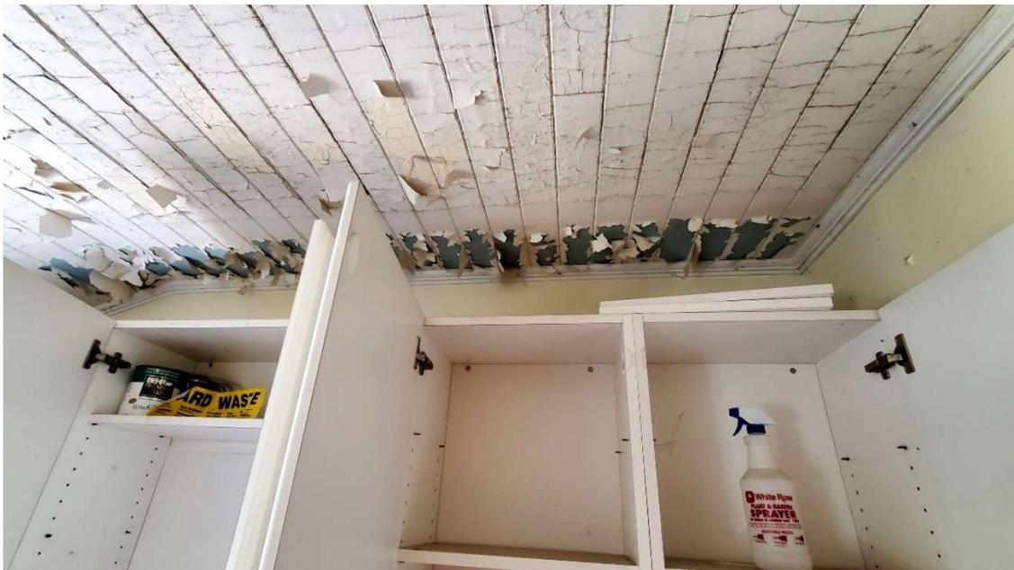
Pic. 14: Peeling/Flaking of Paint in Ceiling due to Moisture Penetration in Laundry room of Building 1B
