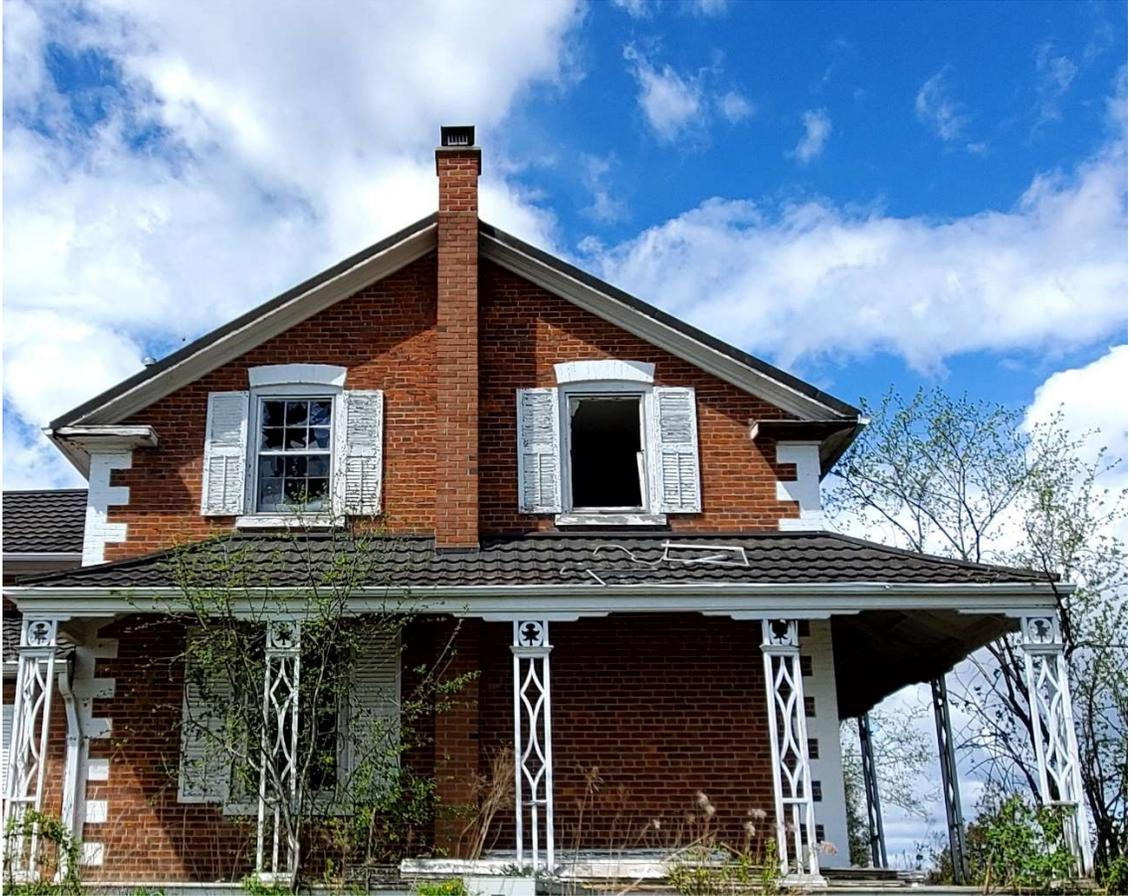
Pic. 39: Degraded Decorative Flat Wooden Posts Supporting Porch and Degraded wood at the Eaves Corner of Roof on Eastside-Building 1A.
