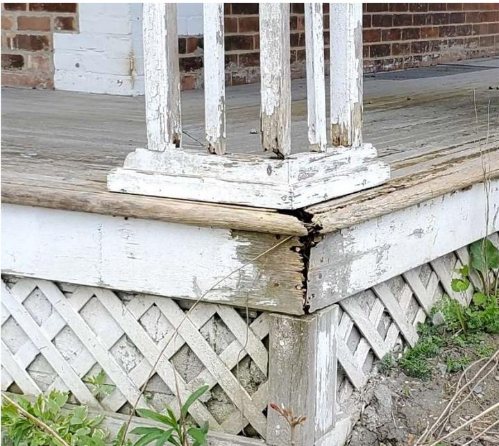
Pic. 41: Compromised Post End, Degraded Perimeter Deck Board of Porch, Covered Deck Floor Structure – Building 1A
