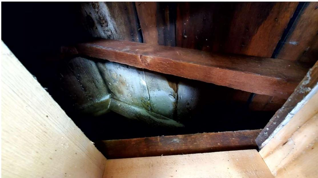
Pic. 49: Wooden Planks on Wooden Rafter – Building 1B
