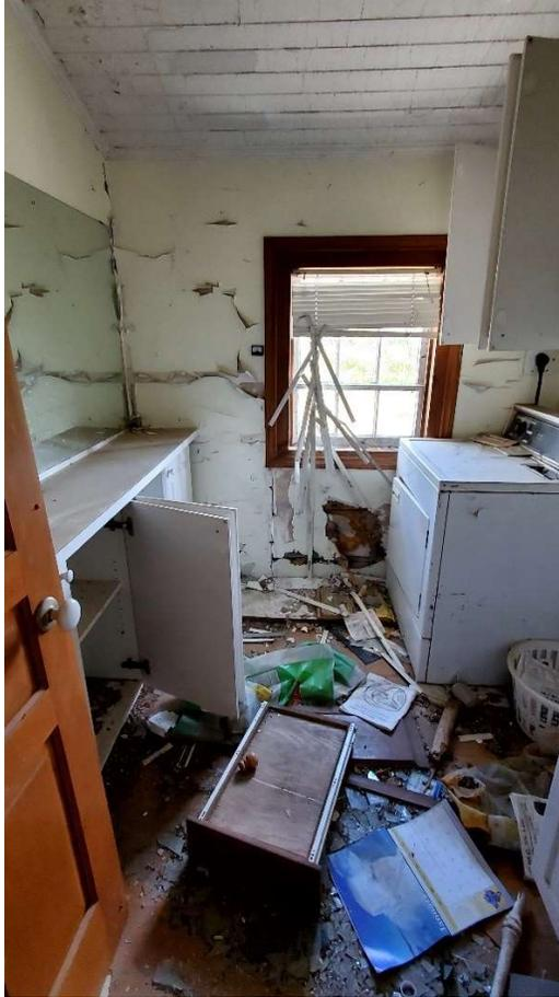
Pic. 13: Laundry in Building B; Debris, Peeling/flaking of Paint and Damaged Wall-Building 1B
