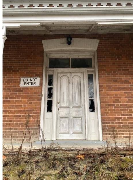
Detailed view of main front entrance, located on the North elevation. Also visible in this photo is the Flemish Bond brick pattern only used on the North elevation of the original farmhouse. The east, west and south elevations of the original farmhouse use a Common Bond brick pattern.
