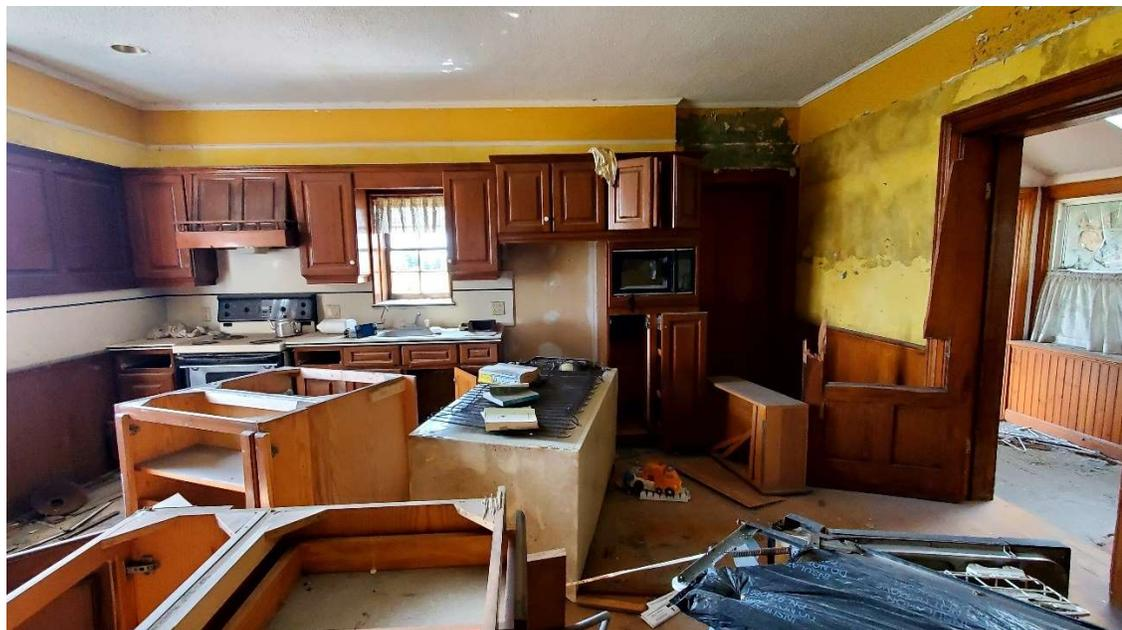
Pic. 10: Kitchen in Building 1B; Penetration Damp on the Walls
