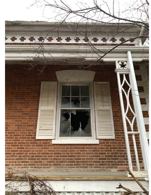
Detailed view of typical window in the original sections of the farmhouse. These windows are original wood double hung windows in a 6-over-6 pattern with single glazing. Aluminum-framed storm windows were added later to these windows and false shutters sit on either side. Shutters were added on later and are not original.
