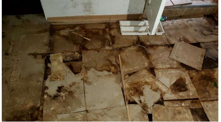
Pic. 37: Water Damaged Stained Flooring over Wooden Floor in Basement of Building 1A
