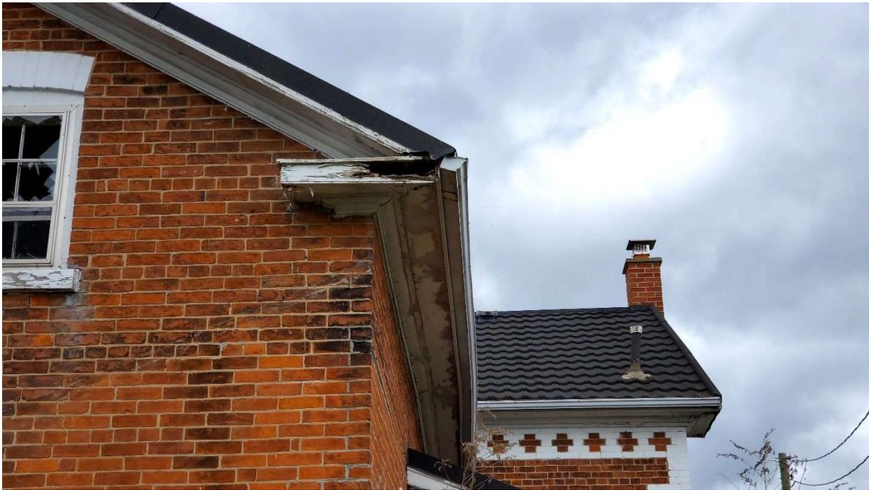
Pic. 38: Previously Repaired Diagonal Crack on Masonry Wall Southside of Building B and Rotten wood at the Eave Corner-Building 1B
