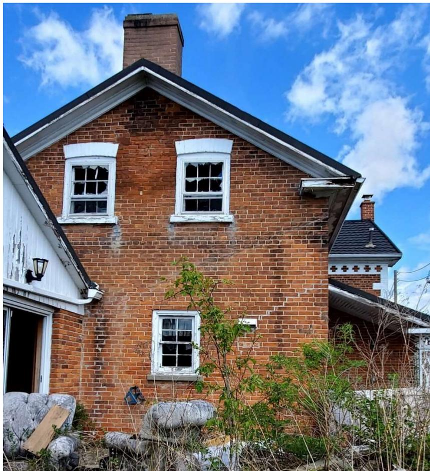
Pic. 8: Southside View of Building 1B– Diagonal crack repairs, watermarks on Brick Masonry Wall, Broken Windows Pane and decayed wood at corner of the eave return.
