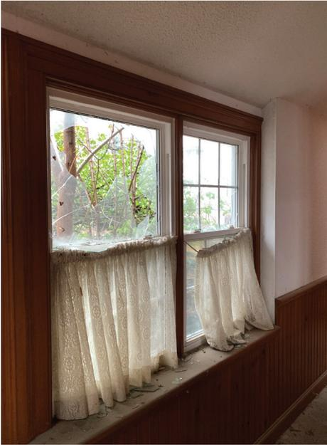
*View of window in the later addition to the south. The windows in this area are 6-over-6 double hung in keeping with the original windows, but they are vinyl windows with double glazing.*
