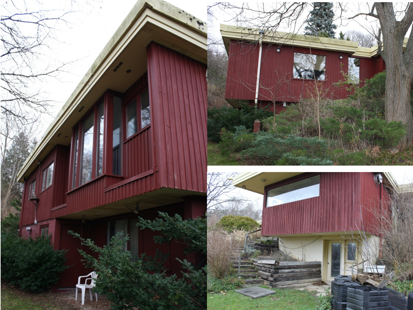
examples of extended cantilever (2012)
