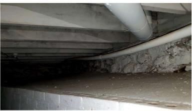
Pic. 31, Pic. 32: Wooden Floor Beam Supported on Rubble Stone Masonry in Basement Crawl Space room-Building 1B
