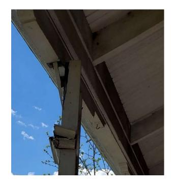
Pic. 46: Damaged Porch Post at Top-Building 1A
