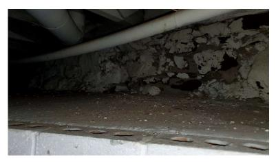
Pic. 29: Patch Work on Rubble Masonry Foundation Wall-Building 1B Basement
