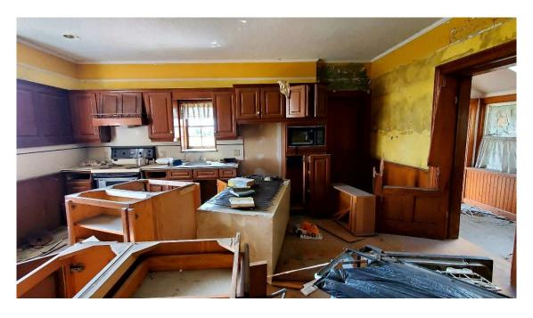
Pic. 10: Kitchen in Building 1B; Penetration Damp on the Walls
