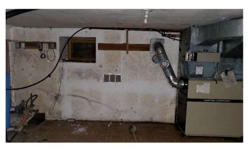
Pic 35: Basement Utility Room, Window, Damp Patches on Exterior Wall-Building 1A
