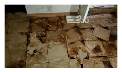
Pic. 37: Water Damaged Stained Flooring over Wooden Floor in
