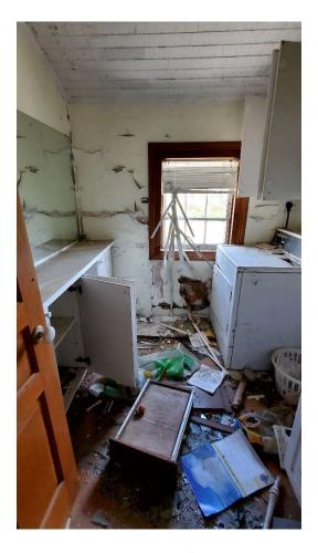
Pic. 13: Laundry in Building B; Debris, Peeling/flaking of Paint and Damaged Wall-Building 1B
