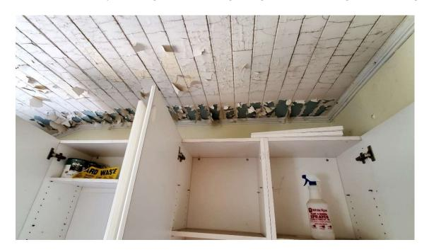
Pic. 14: Peeling/Flaking of Paint in Ceiling due to Moisture Penetration in Laundry room of Building 1B
