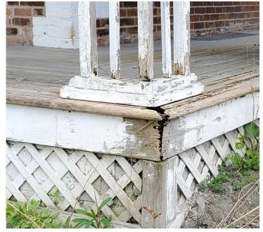
Pic. 41: Compromised Post End, Degraded Perimeter Deck Board of Porch, Covered Deck Floor Structure – Building 1A
