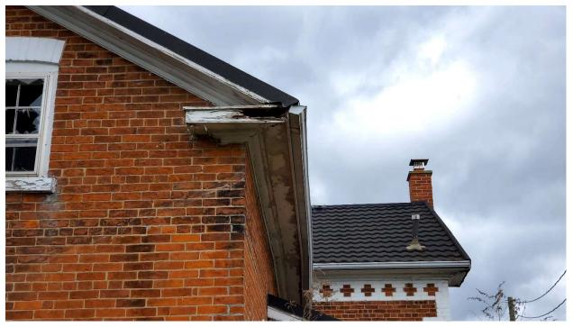
Pic. 38: Previously Repaired Diagonal Crack on Masonary Wall Southside of Building B and Rotten wood at the Eave Corner-Building 1B
