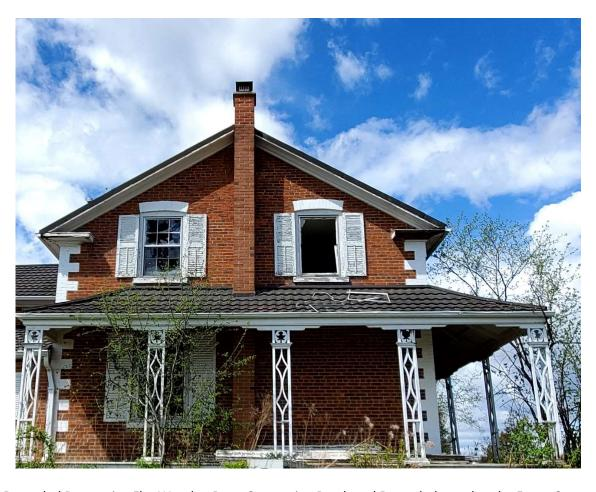
Pic. 39: Degraded Decorative Flat Wooden Posts Supporting Porch and Degraded wood at the Eaves Corner of Roof on Eastside-Building 1A.
