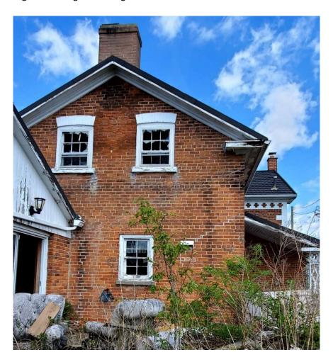
Pic. 8: Southside View of Building 1B– Diagonal crack repairs, watermarks on Brick Masonry Wall,
