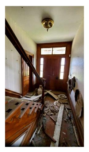
Pic. 21, Pic. 22: Central Corridor with Front Entrance, Stairs leading to the SF with Missing Balustrades-1A
