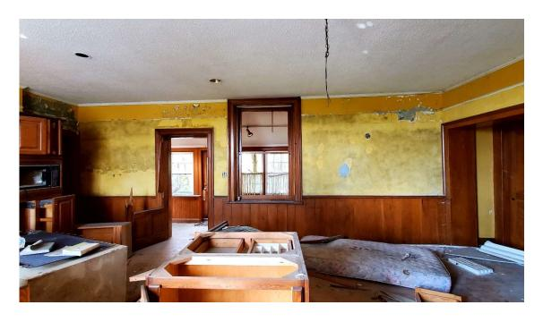
Pic. 11: Westside Wall in Kitchen; Penetration Damp-Building 1B
