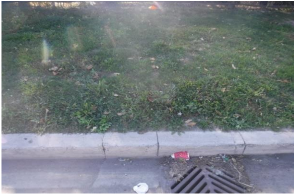
Figure 4.4 Accumulated Large Litter along the curb at the sewer drain
