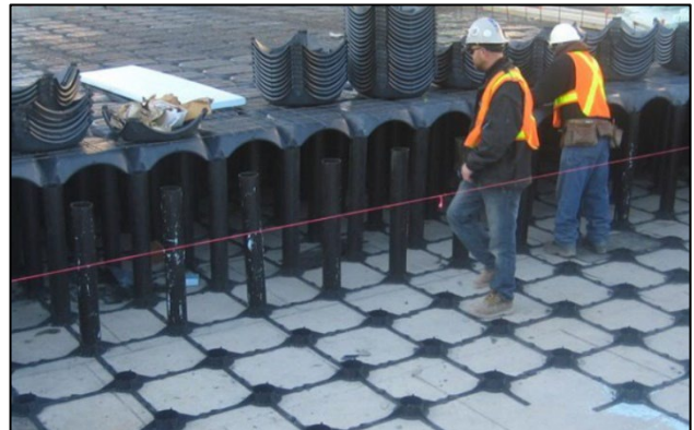
Figure 6: Example Modular Form Cast-in-place Concrete
