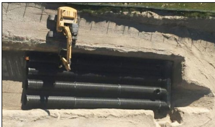
Figure 4: Example of Superpipe System, Source: Contech
