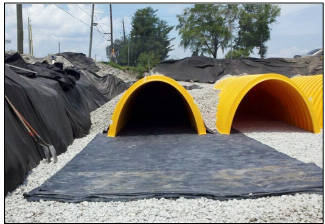
Figure 2: Example of Arch Chamber System, Source: ADS
