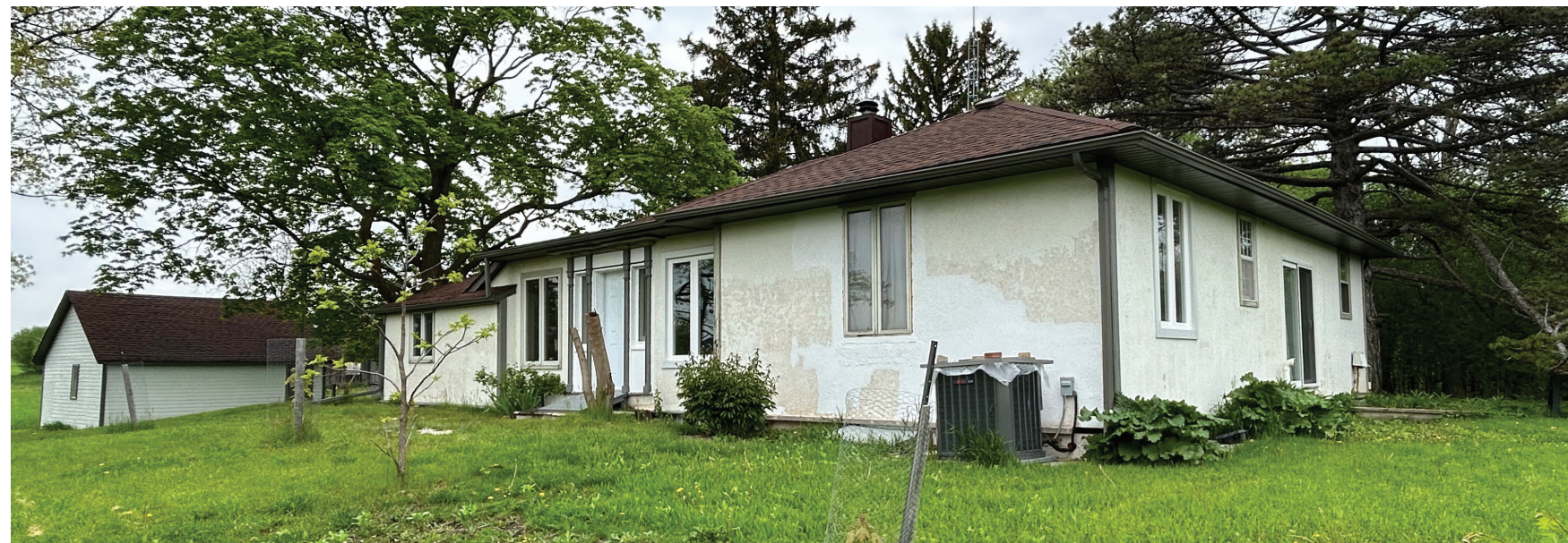
Main House (ERA, May 2024)
