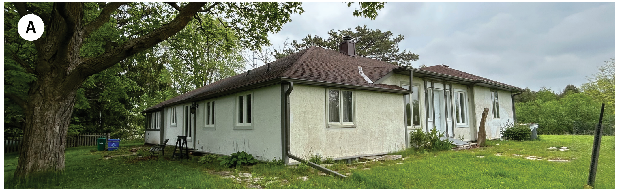
Main House (ERA, May 2024)
