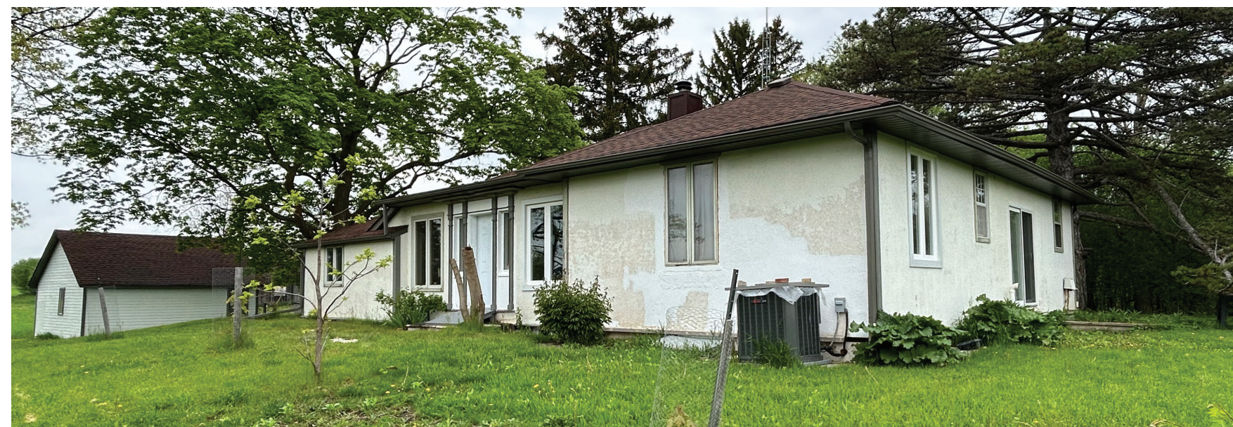
Main House (ERA, May 2024)
