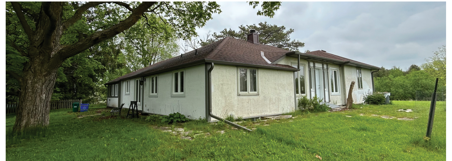
Main House (ERA, May 2024)
