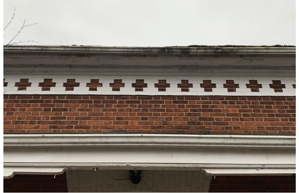
*Detailed view of brick detailing visible on the North and South elevations of the original farmhouse. This is a decorative brick entablature featuring a cross motif.*
