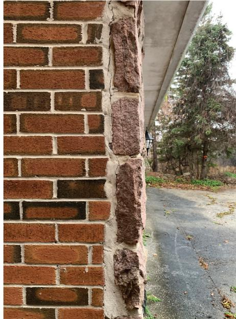
*Detailed view of stone veneer on garage addition. Stone cladding has been stuck. The brick used on the later addition is predominately wire cut brick (seen here) with some hand molded brick on the east elevation.
