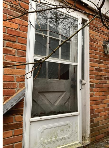
Detailed view of a typical door on the later additions, with an aluminum screen door. Note that none of the doors or windows in the rear addition have brick arches.
