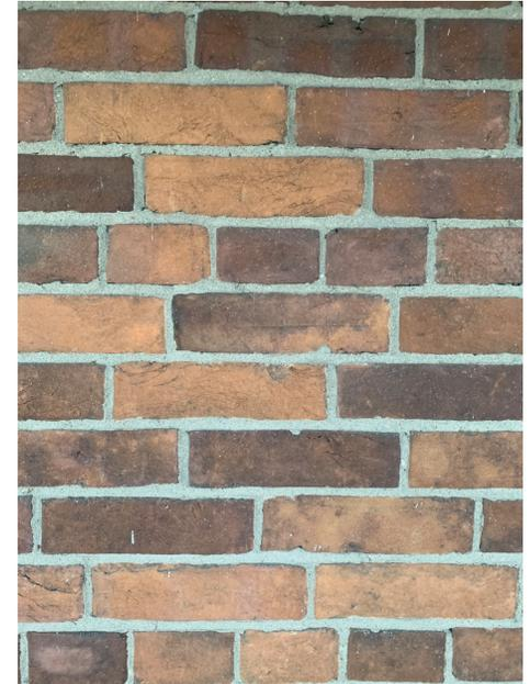
*Detailed view of the brick detailing on the East, South and West elevations of the original sections of the house. As can be seen here, a Common Bond pattern of hand molded brick is used.
