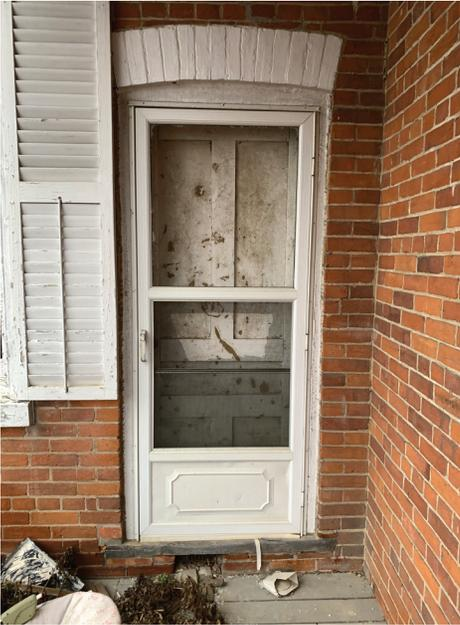
Detailed view of the front entrance, located on the East elevation. Also visible in this photo is the brick arch above the door. These brick arches can be seen over all of the doors and windows in the original sections of the farmhouse.
