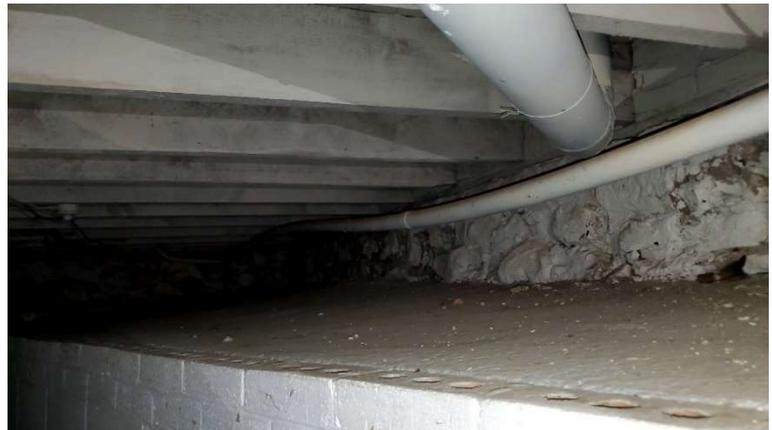
Pic. 31, Pic. 32: Wooden Floor Beam Supported on Rubble Stone Masonry in Basement Crawl Space room-Building 1B
