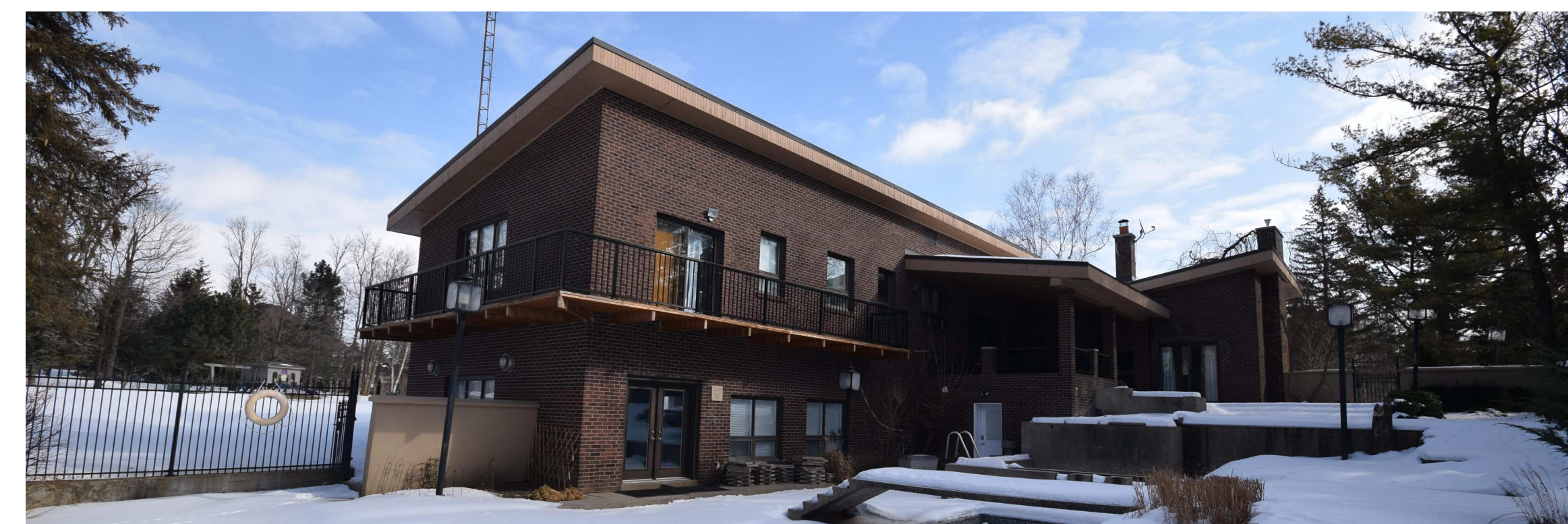
EXISTING REAR LEFT VIEW
