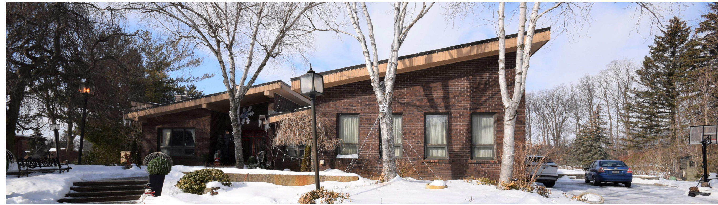
EXISTING FRONT VIEW
