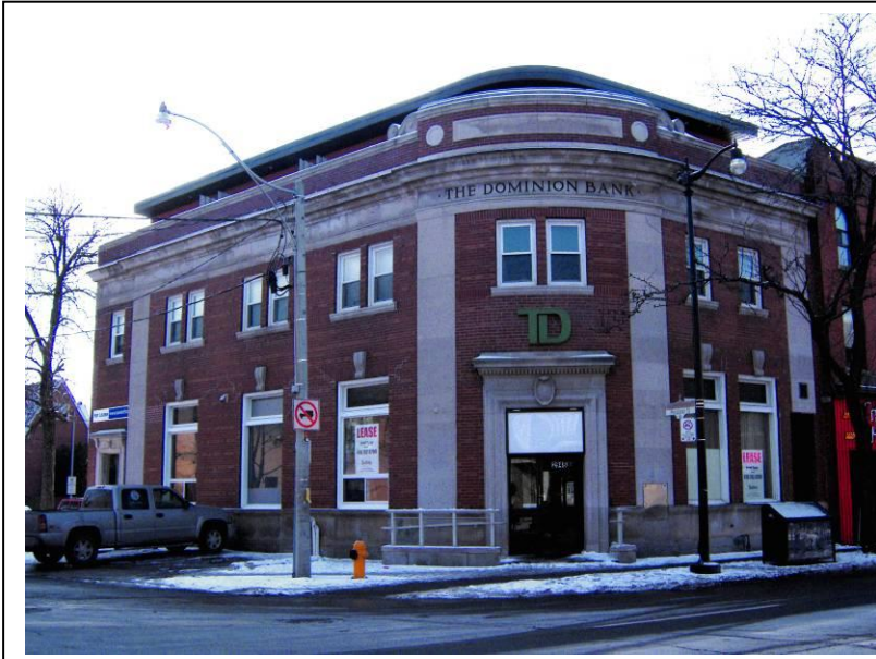
Setting back the third-floor addition allowed the restored bank building to retain its street presence, and maintain the detail significance of the cornice and entry-bay decoration. Preservation Services provided oversight for work under the façade improvement program.
