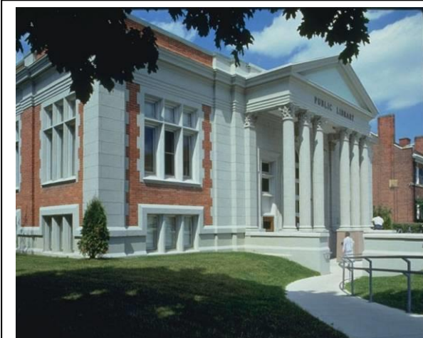
Woodstock Public Library. Phillip Carter's project combined sensitive alterations and an addition with the restoration of one of Ontario's finest Carnegie libraries.
