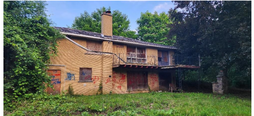
Figure 23 - The rear elevation of 10402 Islington Avenue showing the buff brick, walk out basement, upper balcony and large chimney. (RHC June 2023)
