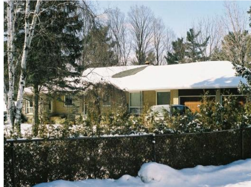
Figure 20 - 10402 Islington Avenue in the winter while the building was occupied. The buff brick accented with Angle stone can be seen as well as paneled wood garage doors (KNHCD Inventory updated Sept. 2021)
