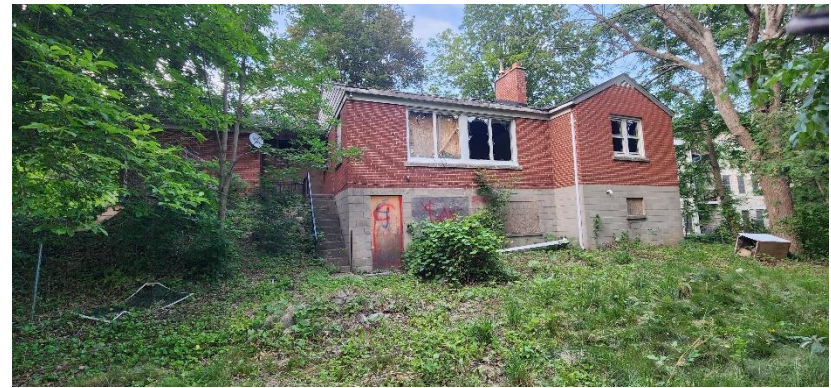
Figure 19 - 10398 Islington Avenue showing the walk out basement at the rear of the building constructed in concrete block. (RHC June 2023)
