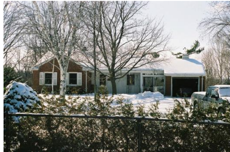
Figure 17 - 10398 Islington Avenue in winter while occupied. In this image the original breezeway between the house and garage has been closed in with sliding glass doors to form a room. (KNHCD Inventory updated Sept. 2021)
