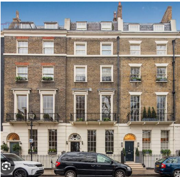
Figure 32 - Examples of Georgian townhouse design in London, UK that illustrate the urban style of Georgian town house as well as the architectural window hierarchy referred to in this section of Recommendations. (Images: Foxtons)
