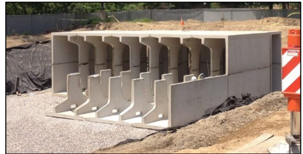
Figure 3: Example Modular Concrete Chamber, StormTrap
