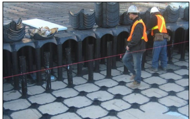
Figure 6: Example Modular Form Cast-in-place Concrete
