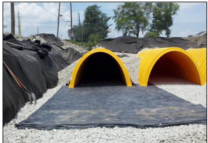
Figure 2: Example of Arch Chamber System, Source: ADS
